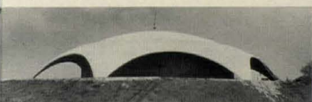
Valley View Reservoir, Lafayette, California. East Bay Municipal Utility District. Designers: Cornelius Sampson and Associates.
