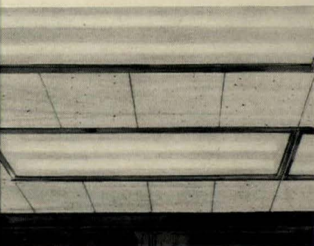
Conventional Lighting System No. 1 (1A) 24" x 48" shielded, recessed troffers—each using one 48" cool white lamp. (Coefficient of Utilization at Room Ratio 5.0, 30% Floor Reflectance, 50% Wall Reflectance: .60)
