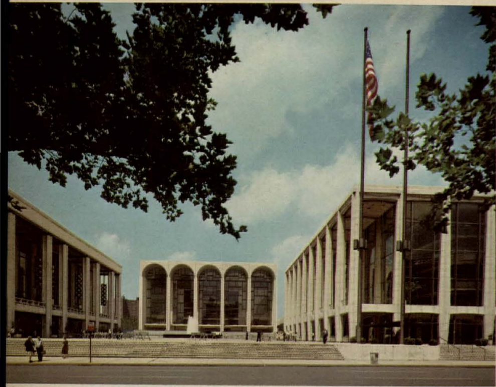
Exteriors of the new opera house: above, as axial focus of the principal plaza; below, in side view; opposite, as seen from the promenade terrace of Philharmonic Hall.
