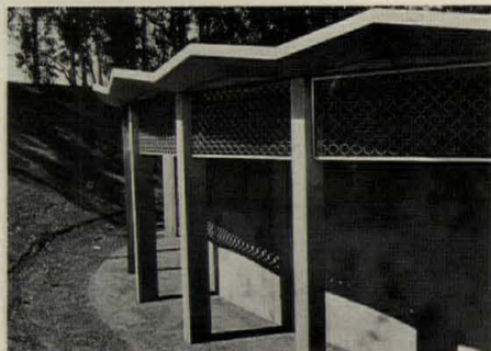
Stanton Reservoir, San Leandro, California. East Bay Municipal Utility District. Architects: Anderson, Hyde, Anderson.
