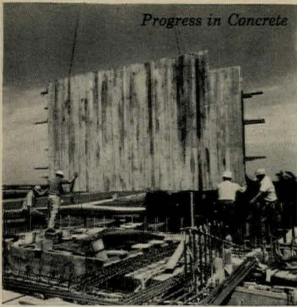
SYMONS STEEL-PLY FORMS GANGED AND LINED
