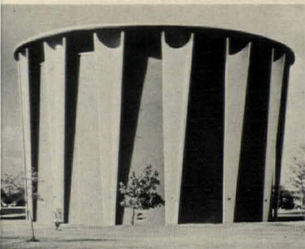
Shadle Park Reservoir, Spokane, Washington. Engineers: The City of Spokane Public Works Department.
