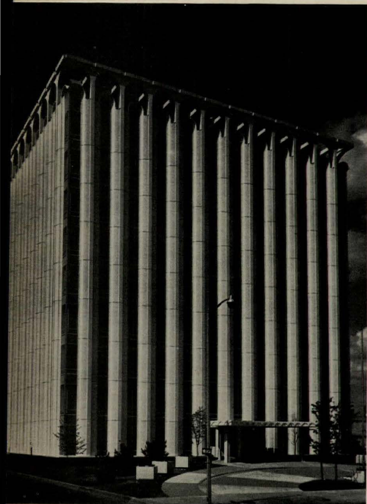
GARVEY CENTER BUILDING, Wichita, Kansas. Architect: S. S. Platt and Associates. General Contractor: Coonrod, Walz and Vollmer Construction Co., Inc. Three Dover Geared Elevators installed by Dover Elevator Co. Group Computamatic® control; speed 350 FPM; capacity 3000 lbs.
