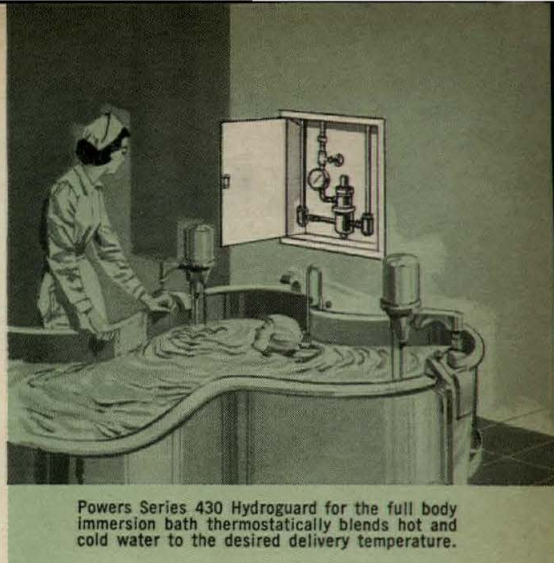
POWERS CABINET SUPPLY FIXTURE Combines a Series 420 or Series 430 Hydroguard thermostatic water mixer, volume control and shut-off valve, dial thermometer, vacuum breaker and recording thermometer alarm unit.
