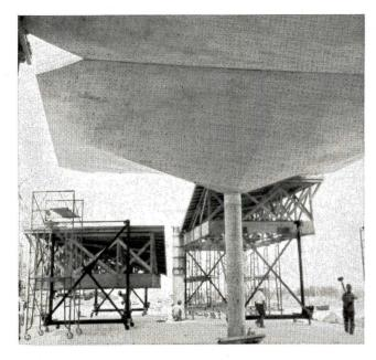
As soon as a completed concrete shell was cured to satisfactory strength, forms were lowered on mobile jacks, rolled to another bay, and raised into position so reinforcing steel could be placed for the next shell. Only 1 hour—often less—was needed to remove both halves of a form from a completed shell and snug them into place around the column at the next bay.
