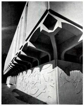
(8) West facade of building features sculptured, cast-inplace exterior walls. (9) Precast panels are used for walls above first floor levels.
