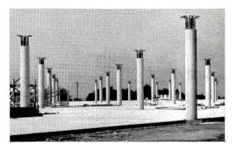
Reinforced concrete columns, 24 in. in diameter, were cast in steel forms using 4,000 psi air-entrained concrete. Designed into each column are electrical conduit and a 4-in.-diameter pipe to handle drainage for the 1,764 sq. ft. shell unit it supports.
