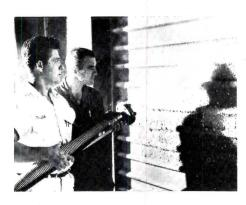
SPRAY-ON INSULATION / K-13 has a UL flame spread rating of 20, fuel contribution of 10, and smoke development of 0 and is thus rated as non-combustible. It has a thermal conductivity K factor of .126563. The insulation is applied by means of a specially designed nozzle which applies both the fibrous material and liquid adhesive simultaneously in separate streams. K-13 adheres to any surface, and has been found to have good sound absorption qualities. ■ National Cellulose Corporation, Houston.
