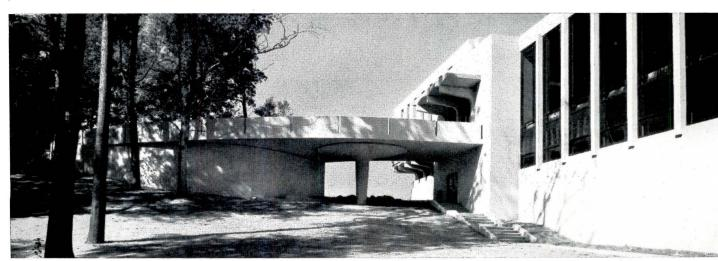
(2) Cast-in-place, post-tensioned entrance bridge takes advantage of the terrain. Bridge was cast integrally with the giant mushroom base. (3) Precast columns are used
