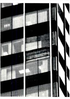
On a gusty March day last year, the wind, whistling around the corner of this New York skyscraper, ripped off the interlocking spandrel panels and sucked out the glass at these corner windows on the 18th and 21st floors.
