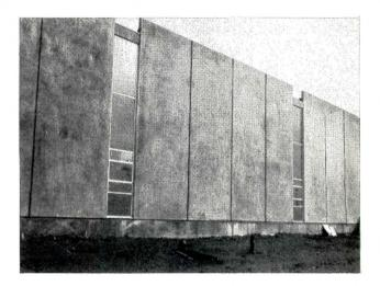
Tilt-up walls offered not only construction economy, but an efficient way to provide for future plant expansion. In addition, they permitted design harmony with the roof. Panel interiors have 1½-in. rigid insulation faced with cement-asbestos paneling. Exteriors are smooth-finished and painted white. Concrete's inherent resistance to fire, weather and abuse assures essential safety and low upkeep cost.
