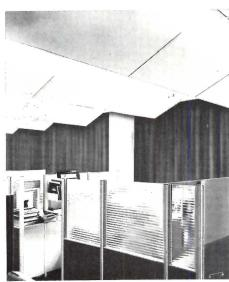
GRID SYSTEM / Acoustical ceiling installations have module, depth and profile flexibility with the 3D Iso-Matic Grid System. The system uses the same standard-size acoustical panels, air diffusers and lighting fixtures as with ordinary suspended ceiling installations. In the photo, a 14-ft ceiling became one with improved lighting and lower noise level.
