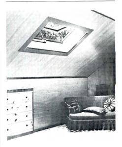
ROOF WINDOW / A leak-proof unit is insulated and provides both light and ventilation. The base is a high-density overlaid plywood. Inner and outer bubbles of the clear acrylic-plastic double dome minimize heat transmission.
