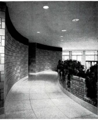
(4) Terrazzo floors add a note of luxury to interiors. (5) Concrete block walls with special exposed surfaces provide decorative effects throughout the structure. (6) Concrete block units are also used in partition walls throughout the building.
