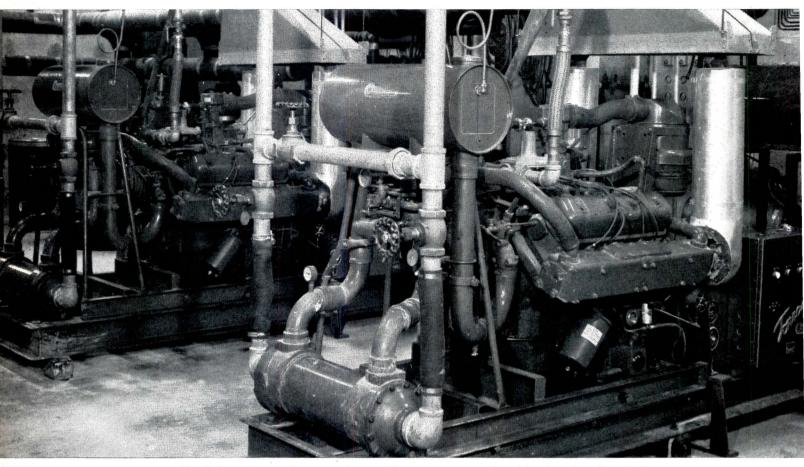
Flexibility of power in a new air conditioning system developed by American Standard permits full conversion of engine power to emergency standby use. This pair of International UV-549's has the set-it-and-forget-it dependability necessary for such a system.
