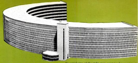
An aerial view of the eight-story semicircular apartments built with standard Spancrete floor and roof planks.
