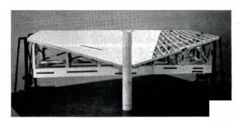
Special roof shell forms, designed and built by the contractor, gave efficient moving and maximum repeat use. 6 sets of forms, each in half-shell sections, were used to cast the entire 88-unit roof. Hyperbolic paraboloid formwork appears difficult to build, yet it is quite simple since the surface is defined by two intersecting systems of straight lines.
