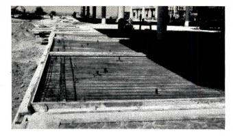
6-in. wall panels, each 26 ft. tall and 19 ft. wide, were conveniently cast right on the plant floor adjacent to their final positions in the wall. When tilted into place, the under side of the panel became the inside face of the wall. The top side, simply screeded and troweled, became the exterior face. 3,000 psi ready mixed concrete of the following mix proportions was used: Type I cement, 470 lb.; water, 240 lb.; sand, 1,465 lb.; 3/4-in. aggregate, 1,921 lb.; entrained air, 5 percent.
