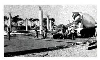
The 6-in. concrete slab-on-ground floor, cast by the checkerboard method, was constructed early in the building schedule. By providing the contractor with a smooth, hard work surface, this speeded moving and shoring of forms and casting of the roof shells. Doing double duty, the floor also served as a casting bed for fabricating of the tilt-up wall panels.
