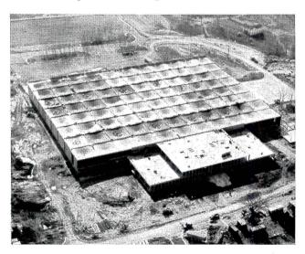
338 by 464 ft. of fully air-conditioned plant space, 65% of the facility's 243,000-sq.-ft. total, is roofed with 88 inverted concrete shells of hyperbolic paraboloid design. Each is 42 ft. sq., 3 in. thick, yet a single column supports it. This roof design offers valuable advantages not only in economy and appearance, but in spacious column-free bays, expanded headroom free of dust-gathering surfaces, improved drainage, along with superior fire resistance.
