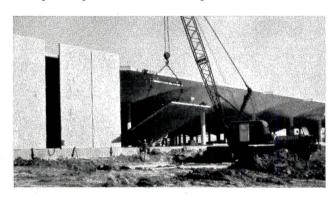
18-ton wall panels were tilted and positioned in as little as 2 hours each with a special telescoping steel strongback devised by the contractor. This was mounted to the panel's upper face and hooked to a crane. The strongback carried two removable jacks with wheels that reached beyond the inner (base) end of the panel, allowing it to roll outward as it was lifted. Once the panel cleared the roof, the wheels were dropped and the panel was turned 180 degrees and fitted to the wall.
