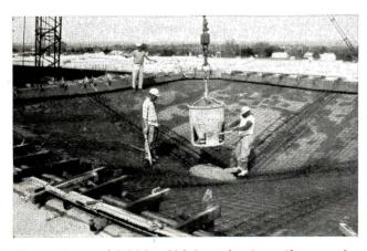
Through use of 4,000 psi high-early-strength concrete, shells were concreted at a 2-per-day rate. Before form removal, specifications required a strength of 3,200 psi, which occurred in 36 to 40 hours with the following mix proportions: Type III cement, 564 lb.; water, 267 lb.; sand, 1,300 lb.; <sup>3</sup>/<sub>4</sub>-in. aggregate, 1,890 lb.; entrained air, 6 percent.
