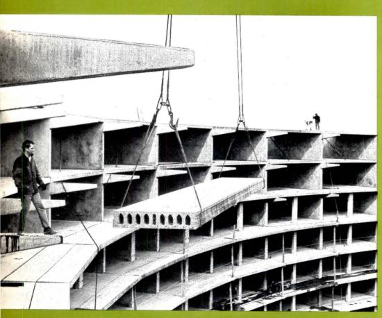
(Top) An 8-inch-deep hollow-core Spancrete plank swings into place.
