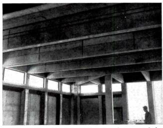
(7) Cast-in-place beams over the recreation area of the building are post-tensioned.
