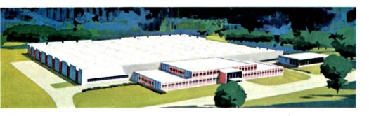
The new office-plant structure of the Monarch Marking System Company near Dayton, Ohio, demonstrates the excitement concrete can bring to industrial buildings. To cover the plant area, architects created a single 3½-acre roof by joining 88 inverted concrete umbrellas 42 feet square, each one self-supporting.
