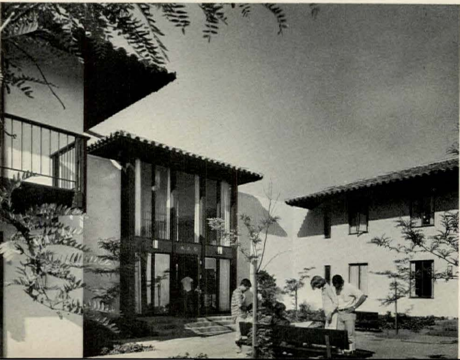
Student Housing Cluster No. 2 at Stanford University by John Carl Warnecke and Associates is organized into a unified yet informal composition which looks inward to its courtyard and at the same time outward toward the campus. The houses are arranged in clusters of three to six units which range from one to three stories in height. This arrangement not only takes advantage of the site, but also eliminates long corridors and facilitates internal circulation. The structures are wood frame with exterior walls of stucco painted in light colors ranging from white to beige. The hipped, red-tiled roofs are part of Stanford's structural vernacular.
