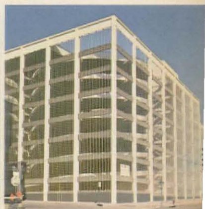
Stadium Parking Garage East, one of 4 multi-level facilities.
