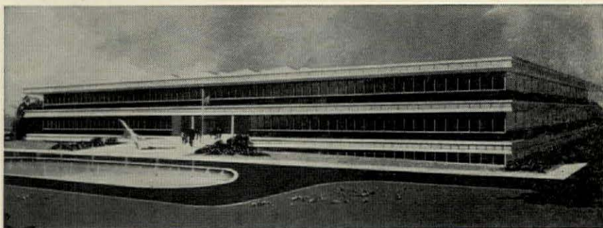
SUNDSTRAND AVIATION GOES VLMC —Sundstrand's 250,000-square-foot, three-story Research and Development Center in Rockford, Illinois, is an outstanding example of the Macomber V-LOK Modular Component System in action. Jones and Brown Company, Inc., represented Macomber in supplying the structural components including steel roof decking. Architects are Larson and Darby, A.I.A. Consulting Engineers are The Engineers Collaborative, and General Contractor is Sjostrom & Sons, Inc.
