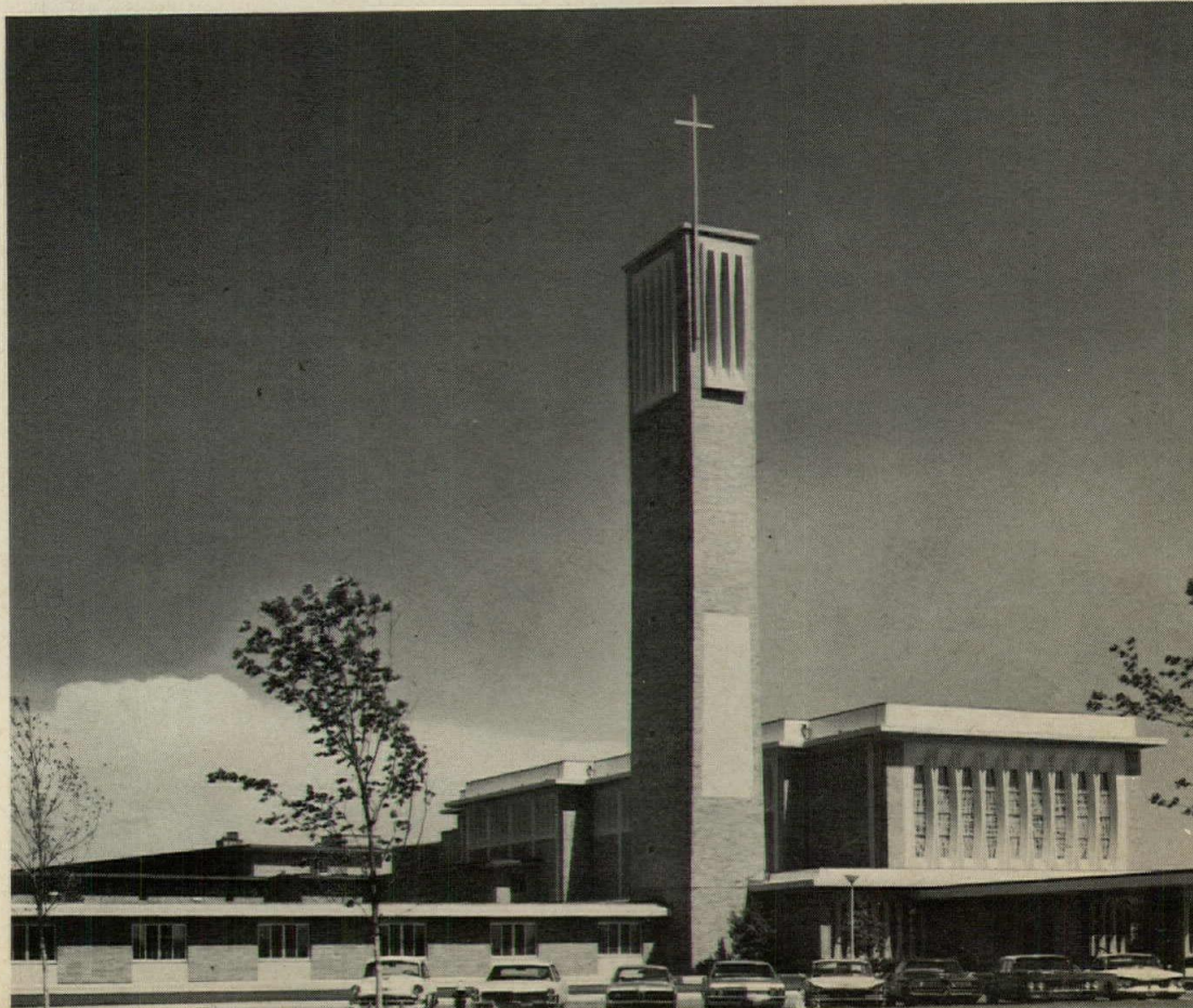
Right: ST. CATHERINE OF SIENA MOTHERHOUSE AND NOVITIATE, Sisters of St. Dominic, Racine, Wis. ARCHITECTS: Barry & Kay, Architects, Chicago. GENERAL CONTRACTOR: Johnson & Herrickson, Racine. Five Dover Oildraulic Elevators installed in various buildings of the complex by Northwestern Elevator Co., Inc., Milwaukee.
