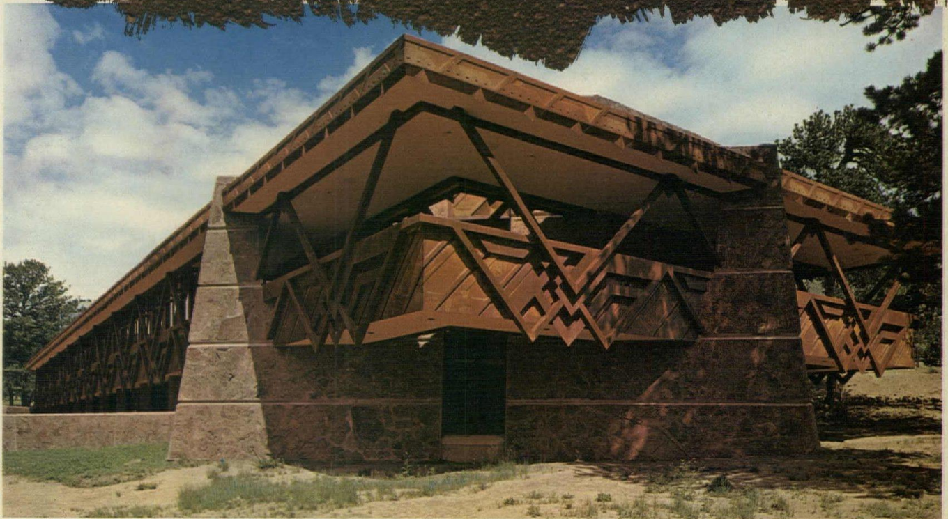
Rocky Mountain National Park Administration Building. Owner: National Park Service, George B. Hartzog, Jr., Director. Architect: Edmond Thomas Casey, Taliesin Associated Architects of The Frank Lloyd Wright Foundation. General Contractor: Kunz Construction Co., Arvada, Colorado. Structural Fabricator: PeCo Steel Corp. (formerly Aladdin Iron & Steel Corp.).
