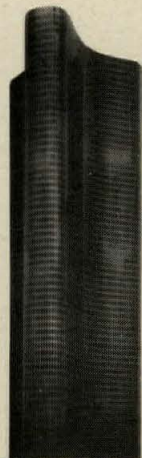
LAKE POINT TOWER Chicago, Illinois Architect: Schipporeit-Heinrich General Contractor: Crane Construction Company Glazing Sub-Contractor: National-Hamilton 1" Polarpane glazing manufactured by Polarpane Corp.
