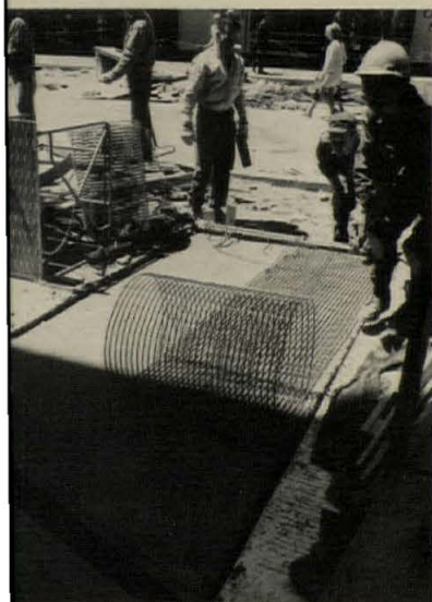
Of various systems being tested, mat to far right (first photo) was ultimately specified. Electrician checks continuity of mat cold lead to splice box connections in sidewalk panel. Next, reinforcing mesh is laid for concrete pour.
