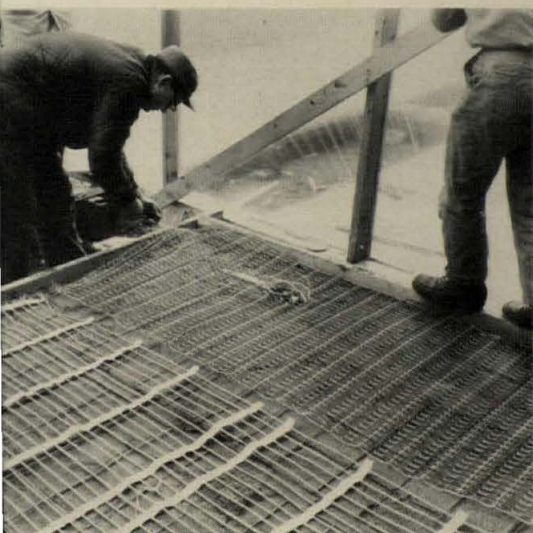
Of various systems being tested, mat to far right (first photo) was ultimately specified. Electrician checks continuity of mat cold lead to splice box connections in sidewalk panel. Next, reinforcing mesh is laid for concrete pour.
