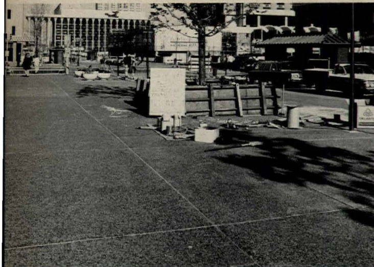
The terrazzo-surfaced mall is divided into snow melting zones, with high wattage mat installations located near stores and at corners for pedestrian
