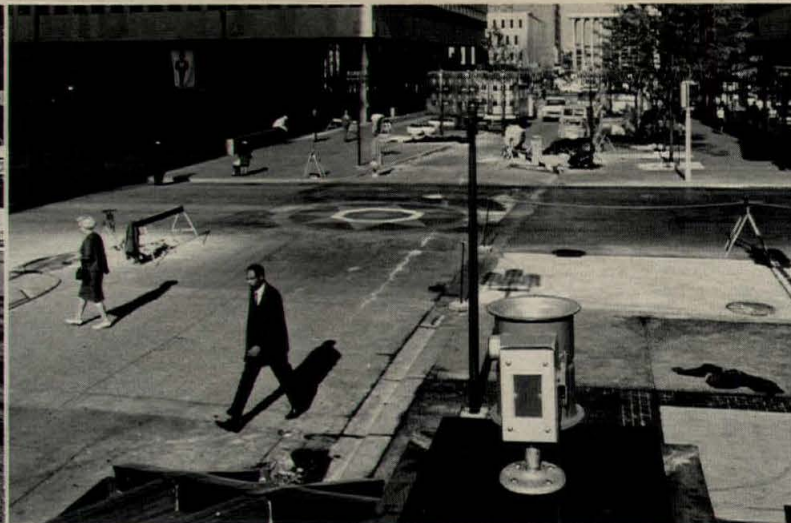
crossings. Snow detector on top of bus shelter, right foreground, activates the melting equipment, set in panels 1½ to 2 in. below grade.
