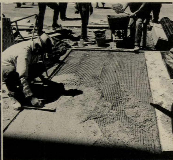
Of various systems being tested, mat to far right (first photo) was ultimately specified. Electrician checks continuity of mat cold lead to splice box connections in sidewalk panel. Next, reinforcing mesh is laid for concrete pour.
