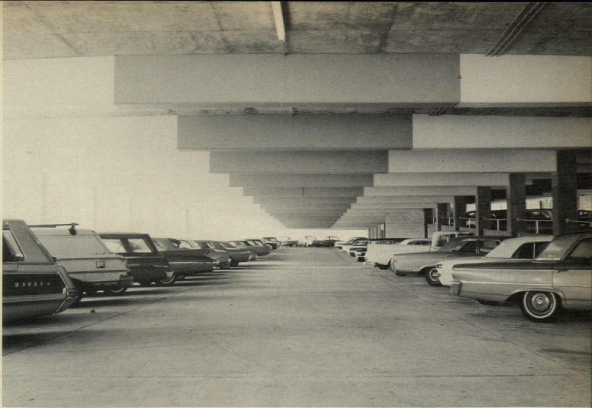
Clear-span construction provides wide drive aisles and easy-angle parking. The beams are color-coded (strip in center) for patron's ease of reference. The exit ramp is of the straight-down type; ramp entrances are shown at two levels.
