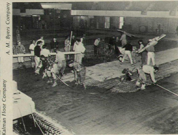
The ice rink is one huge, jointless, concrete slab filled with closely-spaced wrought-iron pipes for freezing the ice. A special slip plane was provided to allow the slab to move freely.
