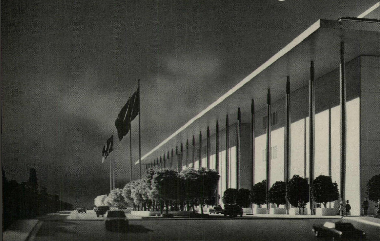
The John F. Kennedy Center for the Performing Arts, Washington, D. C. Edward Durell Stone, Architect
