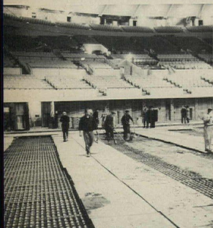
The ice rink is one huge, jointless, concrete slab filled with closely-spaced wrought-iron pipes for freezing the ice. A special slip plane was provided to allow the slab to move freely.
