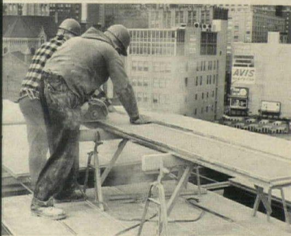
or structure is steel-edged gypsum planks attached to bar joists. Plank edges are welded to the joists and to each other to form a diaphragm. Planks form a working platform for the workmen.
