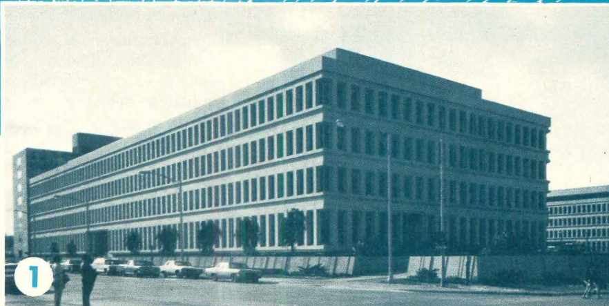
4-Story Office Building of the State Capitol Development Lansing, Michigan.
