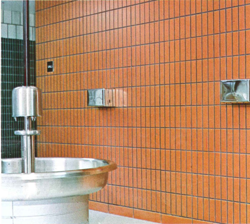
This wall was laid with 8x16 block!
