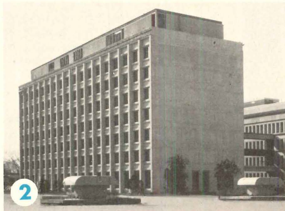
7-Story Office Building of the State Capitol Development, Lansing, Michigan.
