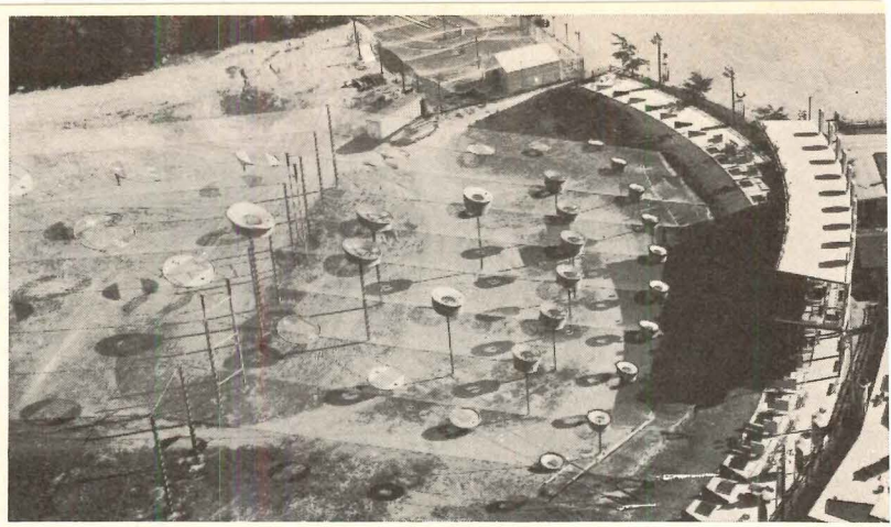
Stargets Golf Course, Hanover, Massachusetts Designer-Owner: Family Leisure, Inc., Engineering Consultant: Simpson, Gumpertz & Heger, Inc., Project Engineer: John F. Notemeyer, Steelwork: Chestnut Welding & Iron, Inc., General Contractor: Taverna Brothers
