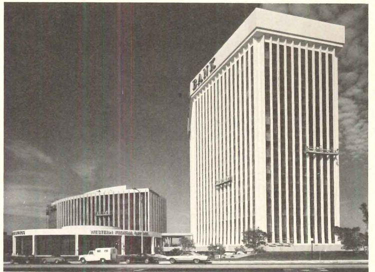
The Del Amo Financial Center, Torrance. Victor Gruen Associates. The project "contains the first modified ductile frame, reinforced concrete high-rise building designed to meet the new seismic code requirements of the City and County of Los Angeles."
