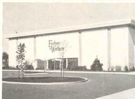
Forbes & Wallace Department Store Designers: Raymond Loewy/William Snaith, Inc. Engineers: Strobel and Rongved, Engineers Herman Blum, Consulting Engineers
