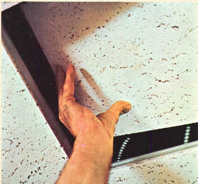
In corporate headquarters offices of Heublein, Inc., in Hartford, Conn., tiles fit snugly in the Accesso Concealed Suspension System to form a smooth, almost seamless ceiling.
