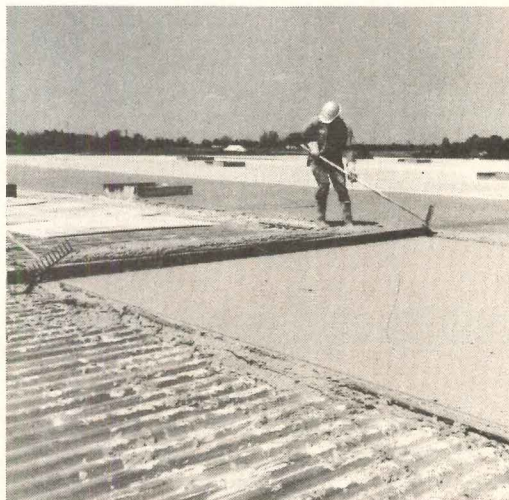
Celramic fill is easy to work, but won't bleed through joints.
