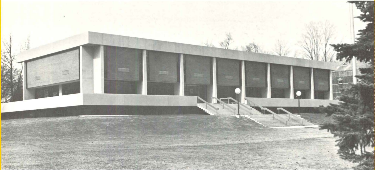
Dean Junior College Library in Franklin, Massachusetts—a handsome addition to the college campus.
