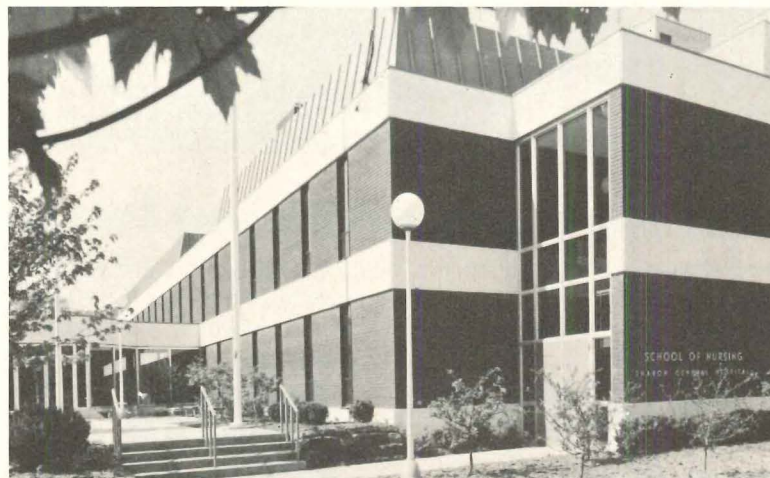
School of Nursing and Morrison Hall, Sharon General Hospital, Sharon, Pa. Architect: Brooks & Redfoot, Sharon, Pa. Sheet Metal Contractor: The Woodward Company, Warren, Ohio Photographs: Frank S. Pavliga
