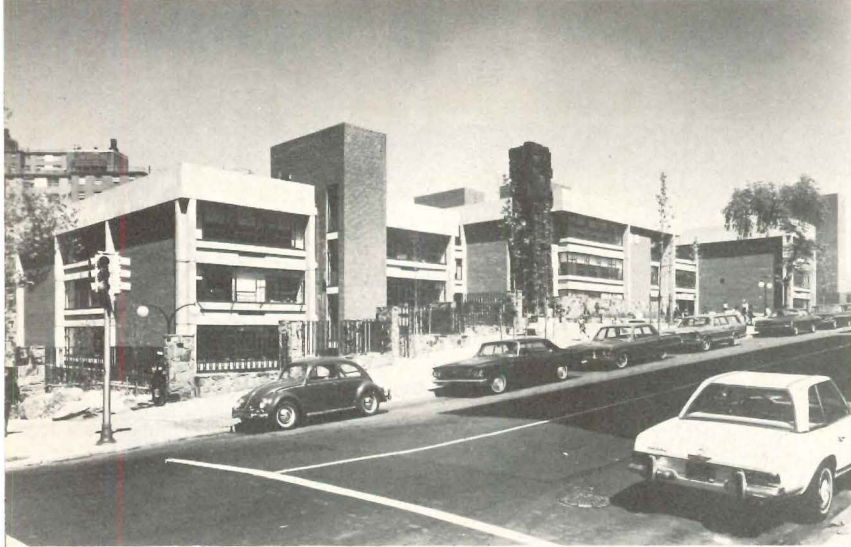
Morningside School (P.S. 36) , Manhattan, N.Y., Frost Associates, architects (November, 1968, page 151) avoids a structure that would dominate small children (aged 5-7) by dividing into three units. Bridges, which serve as lunchrooms and play areas, connect the three separate class buildings to a central administration unit.
