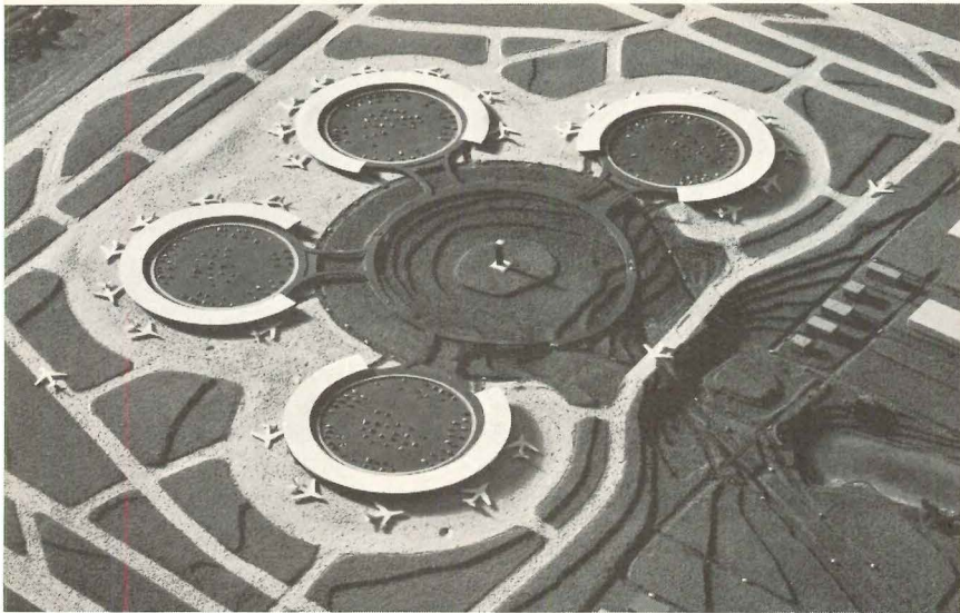
Space-age appearance and efficiency of Kansas City International airport is made possible by extensive use of Grade 60 Steel. Total tonnage of high strength reinforcing steel is 5350 tons.
