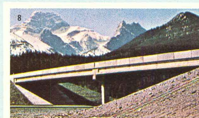
8. PRECAST PRESTRESSED GIRDER BRIDGE 9. TENDONS IN PLACE FOR POST-TENSIONED SLAB
