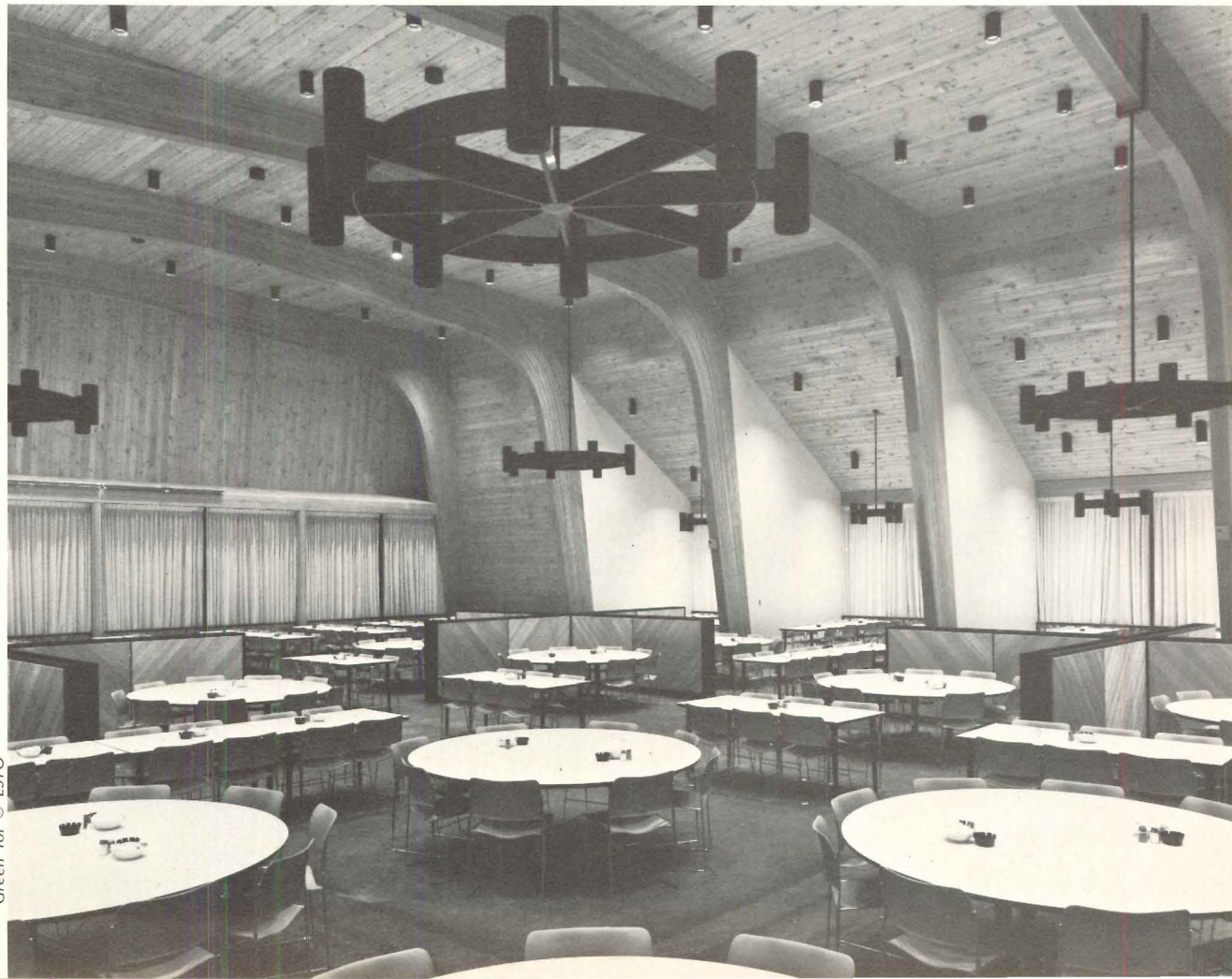
The dining hall (right and below)—another key building—shares its architectural vocabulary with the student activity building and the gym. Wood bent construction has been used to ease footing loads because of poor bearing.
