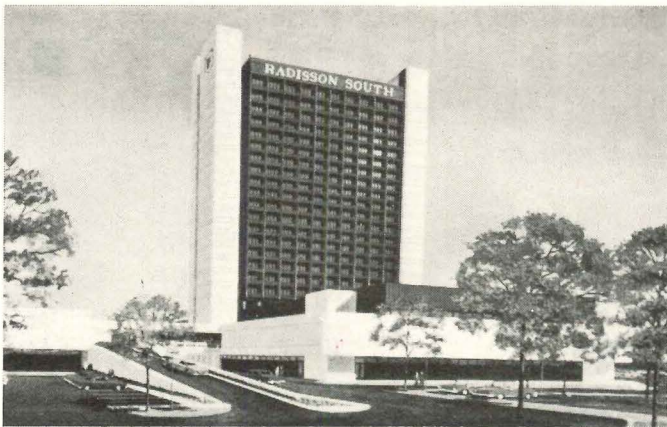
RADISSON SOUTH HOTEL, Minneapolis, Minn. Owner: Radisson Management Association Architect: The Cerny Associates, Inc. Structural Engineers: Intertec, Inc., and The Cerny Associates, Inc. General Contractor: Earnest M. Ganley Construction Co. Fabricator: Paper, Calmenson & Co. Erector: L. H. Sowles Co.
