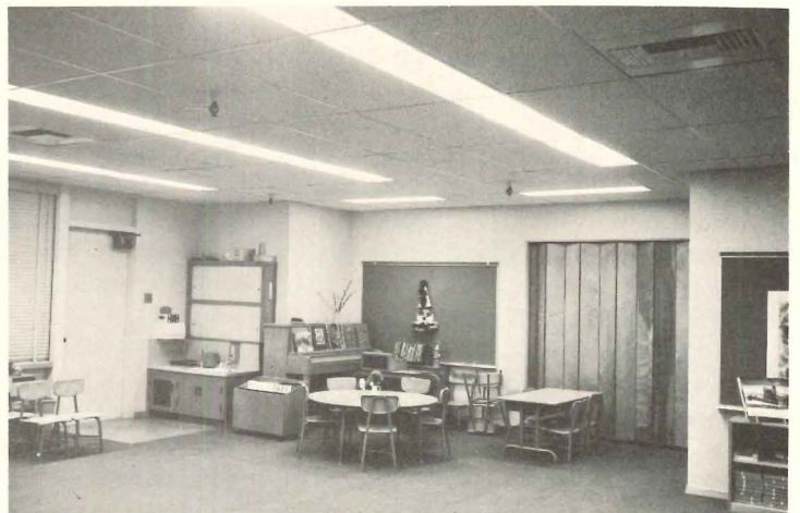
7. Two-lamp, recessed, 12-in. wide, lens panels, in continuous rows, 7 ft on center. LEF = 0.182 CRF = 0.766
