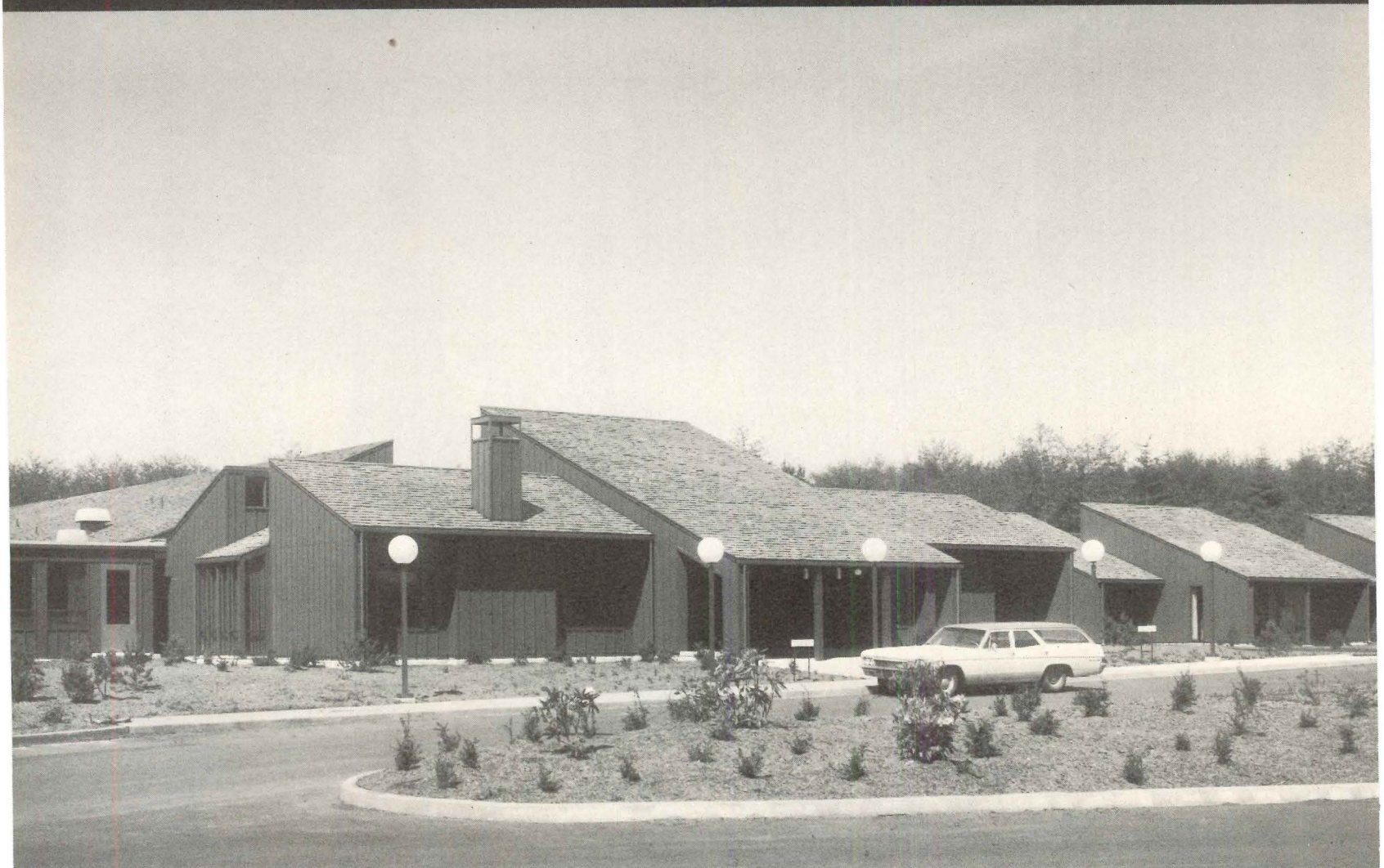
North Lincoln Hospital, Lincoln City, Oregon. Certi-Split No. 1 Handsplit/Resawn Shakes, 24" x 1/2" to 3/4". Architects: Edmundson, Kochendoerfer, Kennedy, Daniel, Mann, Johnson & Mendenhall. Builder: George A. Moore & Associates
