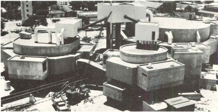
The Mummers Theater , Oklahoma City, Okla., John M. Johansen, architect, is designed to be a loose, functional, free arrangement of components: a large theater, small theater, and rehearsal hall-school, and sub-components: offices, lounges, etc., interconnected by "circuitry systems"; stairs, ramps, bridges. It is meant to provoke and invite the passer-by, and to be, in many ways, a product of chance.
