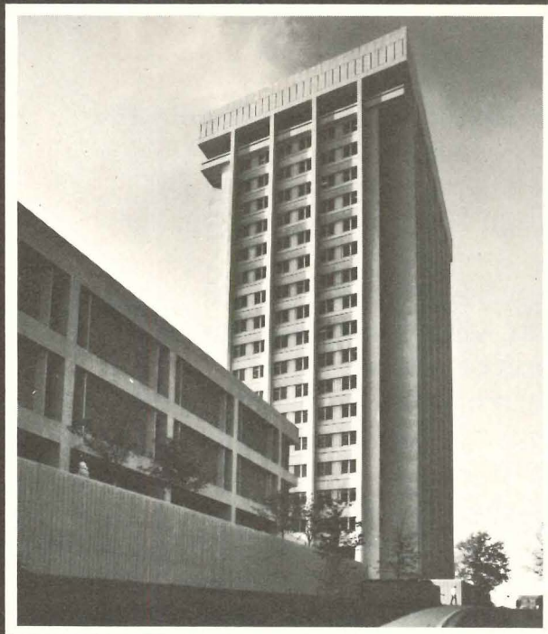
(Above) Patterson Office Tower and White Classroom Building. Architects: Johnson-Romanowitz, Lexington. General Contractor: Foster & Creighton Company, Lexington. Six Dover gearless traction elevators with Computamatic IV Control.
