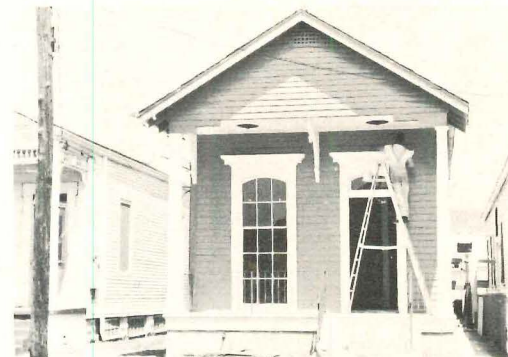
New Orleans In addition to its planning work, Metro Link has been involved in several housing rehabilitation projects. Working with the Archdiocese of New Orleans, the CDC has assisted in the renovation of seven "shotgun" houses in the Irish Channel area, above. Their sturdy cypress structures made them good candidates for rehabilitation. Brother Dan, one of the monks assigned to the project, completes the painting.
