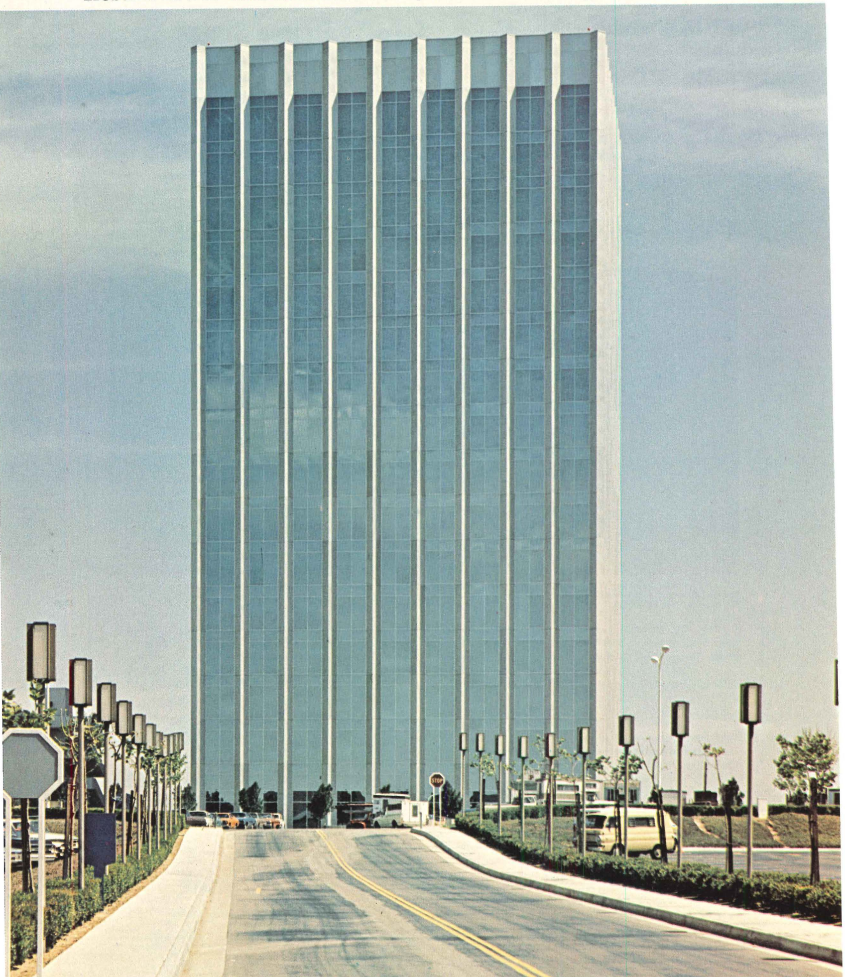
Avco Financial Center, Newport Beach, California. Owner: Balboa Insurance Company • Architects: Welton Becket and Associates • Consulting Mechanical Engineers: James A. Knowles and Associates, Los Angeles • Glazing Contractor: Golden State Glass Company, Los Angeles
