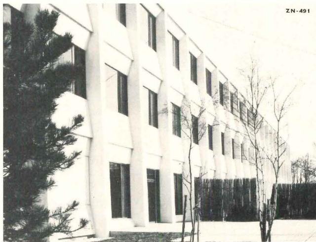
IBM's beautiful Data Processing headquarters utilizes galvanized re-rod to prevent sub-surface rust and consequent staining.
