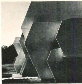
Cover: Burroughs-Wellcome Co. corporate headquarters Research Triangle Park, Raleigh, North Carolina Architect: Paul Rudolph Photographer: Joseph W. Molitor
