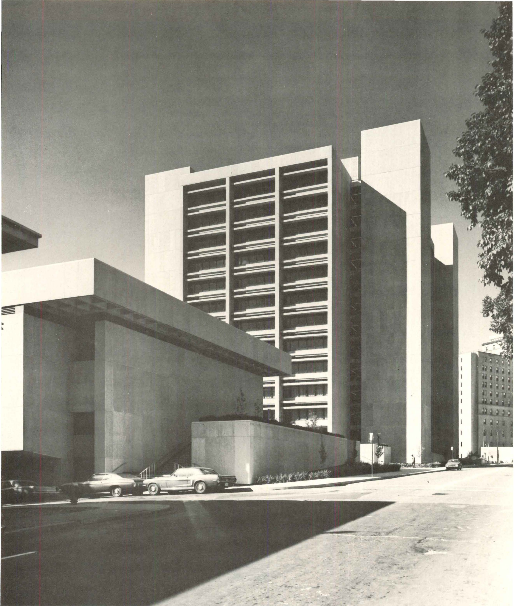
UNIVERSITY OF PITTSBURGH SCHOOL OF ENGINEERING (Michael L. Benedum Hall). ARCHITECTS: Deeter Ritchey Sippel Associates. BUILDER: General State Authority, Commonwealth of Pennsylvania. Dover Elevators installed by Marshall Elevator Co.
