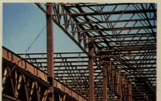
The ease and versatility of designing with steel joists and joist girders solve other-wise complex design problems.
