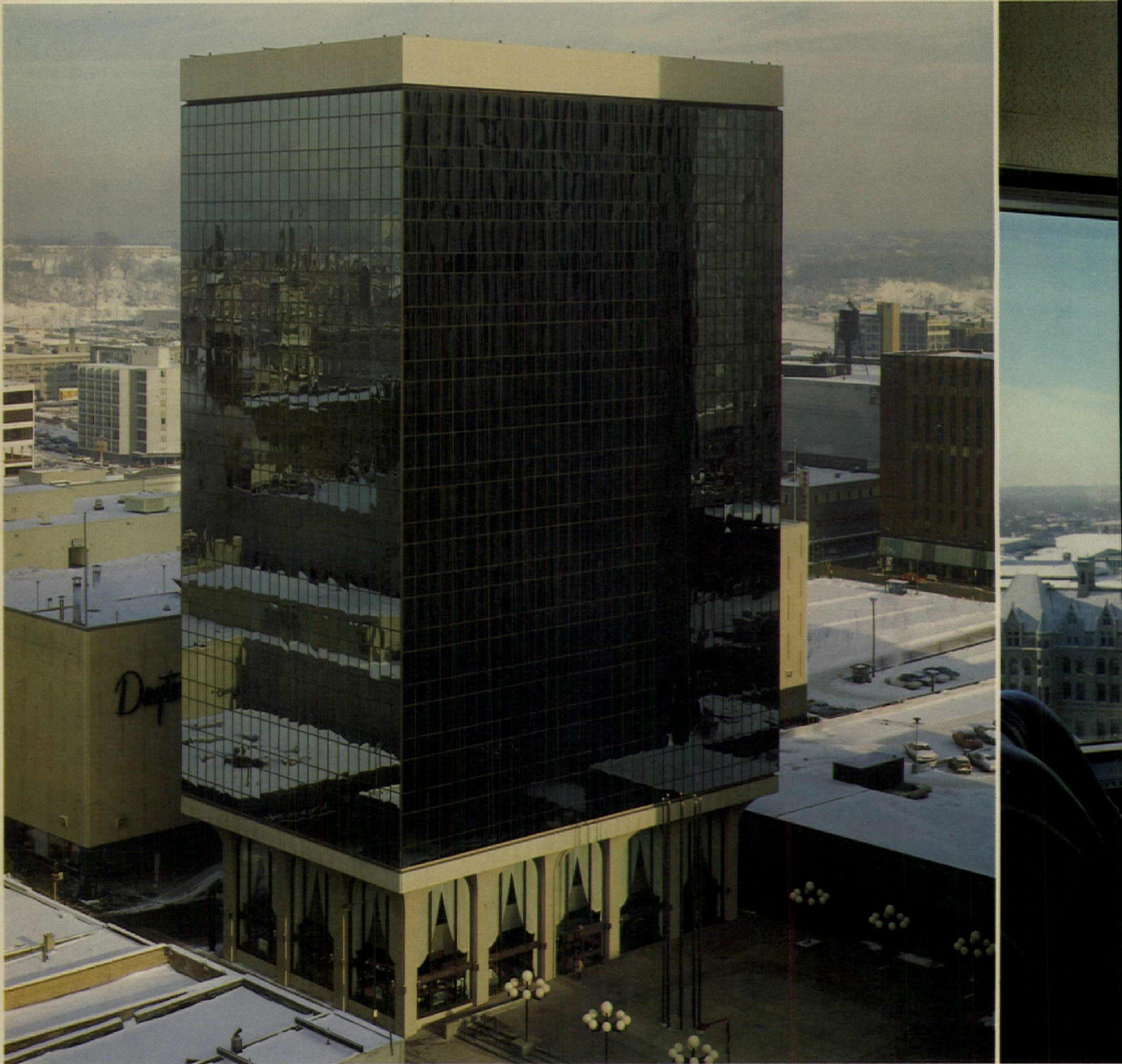
Northern Federal Building, St. Paul, Minnesota. Owner: Yorktown Investment
