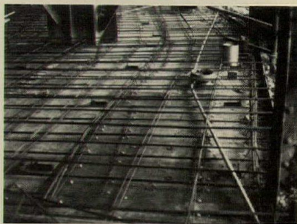
Galvanized rebar under surface of decking.
