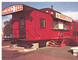
Whistle Stop Restaurant, Phoenix, Arizona, Clarke Modular, Inc., Glendale, Colorado.
