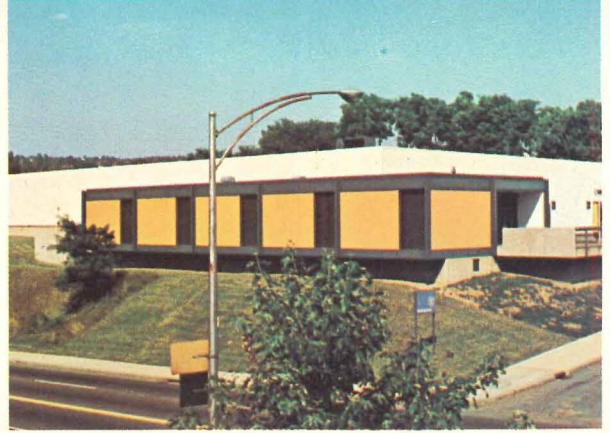
Westinghouse Electric Corporation Homewood Plant, Pittsburgh, Pa. Architect: Walter Roberts Associates, Pittsburgh, Pa. C-Panel System, 4" and 8" Ribbed Exterior Profile.
