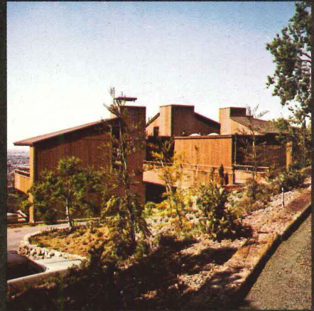
Inverted Batten Ruf-Sawn redwood plywood on custom residence
