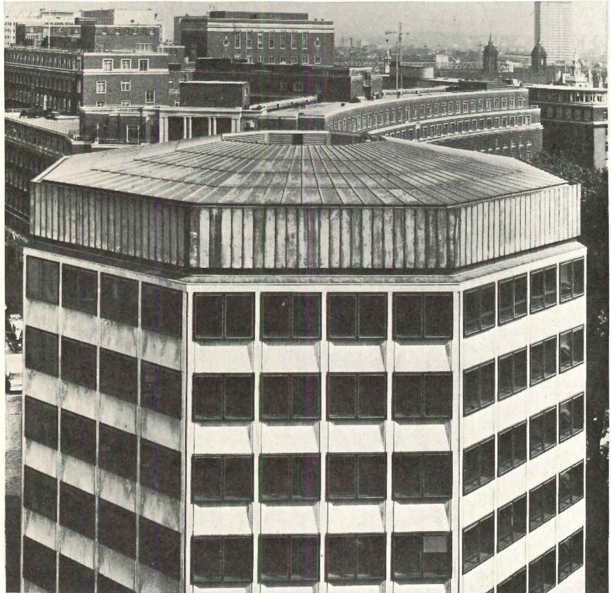
The fascia of the roof of this six-story building is in the form of an open screen comprised of 200 panels of lead clad steel. The panels are fabricated from 20 gage steel with a lead coating of about 1½ pounds per sq. ft. (.0234" thick) on each side.
