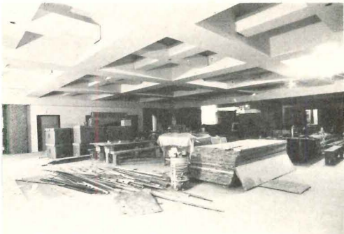
Photo above shows how a basic ceiling pattern can remain exposed in sections where mechanical and electrical requirements and interior finishes do not call for a suspended ceiling.
