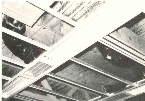
The module of the ceiling grid permits flexible installation of units for both lighting and air distribution at any required position.
