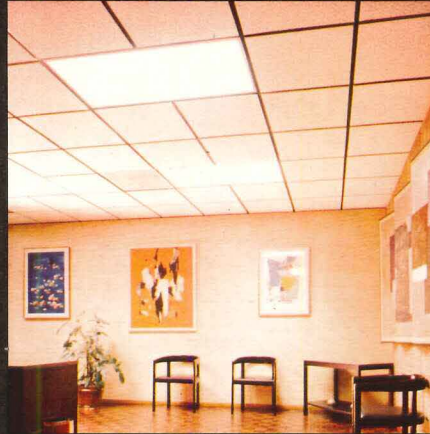
Recessed edge, non-directional fissured Pyrotec ceiling
