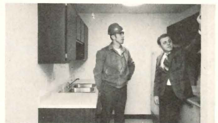
Hide-A-Spray paint dried in two hours. Contractor installed cabinets and floor covering the same day. Walter Scharfe, left, Job Superintendent for Lloyd Construction, commented, “Conventional two-coat paints would have meant a week’s time between painting and any such installation.” PPG Paint Center Manager, Eugene Lee, is shown at right.
