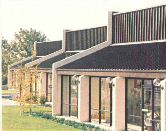
The system permits pleasing roof variety.
