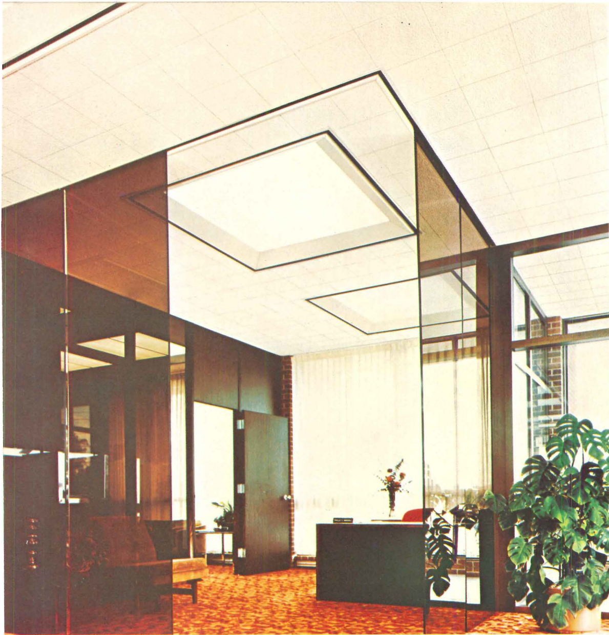
First Federal Savings & Loan Assn. of Danville , Martinsville, Virginia. Architect: Calvert, Louis & Smith. Acoustical Contractor: J. W. Squire Co. Banking area ceiling: Conwed 12" x 12' Rock Face Ceiling Tile.
