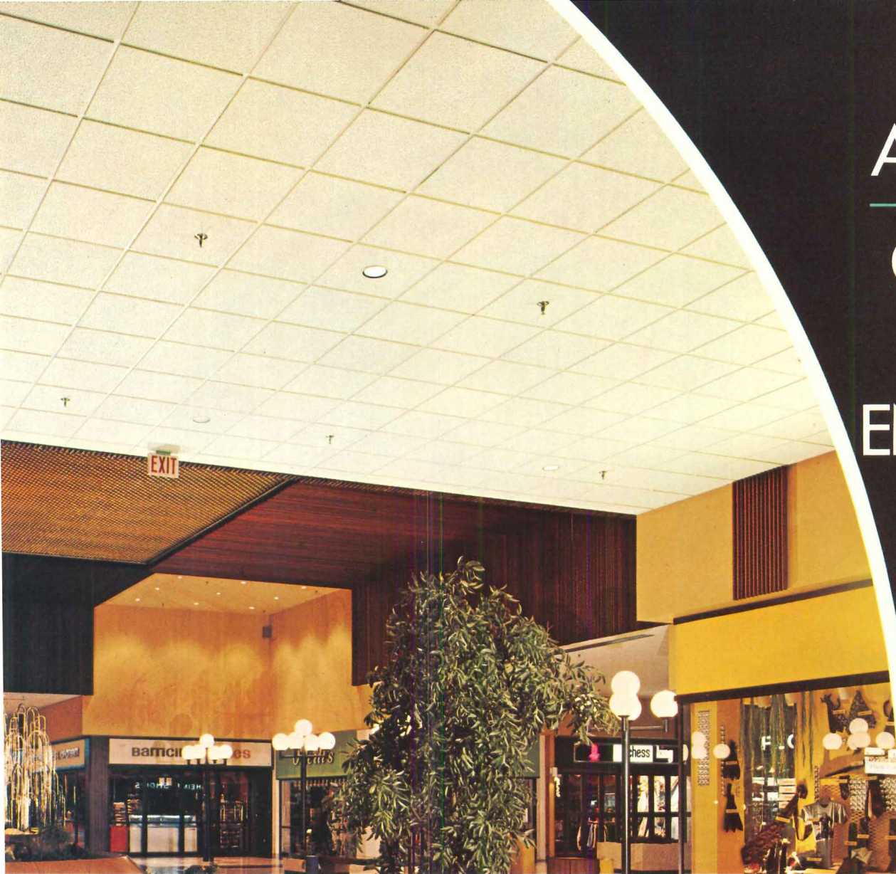
Cloverleaf Mall, Richmond, Virginia. Architect: Carneal and Johnston. Acoustical Contractor: Consolidated Tile Co. Ceiling: Conwed Rock Face 24" x 24" Reveal Panels.
