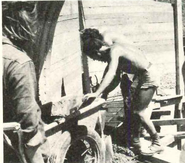
The Restaurant building (below and left) is being completed this summer for use as an eating and reception facility. The majority of its parts were precast, and set-in-place with a crane, which is Arcosanti's sole piece of heavy equipment. Most of the work, however, is done more or less by hand, as in the photo at left. The Ceramic Apse, far left, was silt cast, like the previous buildings.
