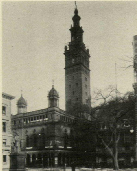
“Madison Square Garden, New York, 1889. McKim, Mead and White; Stanford White, designer. Demolished. Part north Italian, part Spanish, in white terra cotta and pale buff brick; on top of the Giralda-like tower, the second version of Saint-Gaudens' Diana.”
