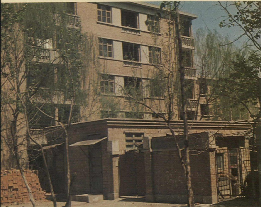
Housing project above in Peking is typical of urban housing throughout the country—four or five stories high, red brick, red tile roofs—with modest decoration in the form of precast balconies or brick corbeling. As soon as a project is completed, the courtyards are closely planted with trees to produce a green, park-like setting.
