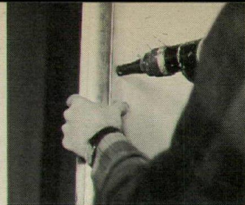
3. Attaching core to T-spline.
