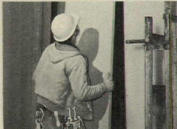
2. Installing core panel.
