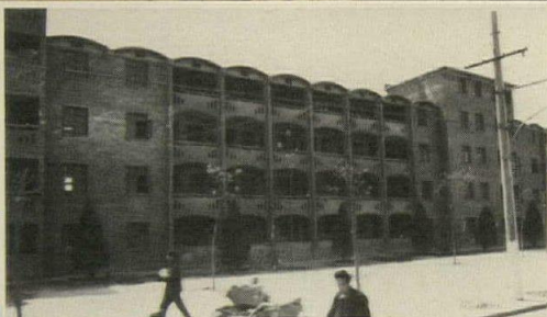
Housing project above in Peking is typical of urban housing throughout the country—four or five stories high, red brick, red tile roofs—with modest decoration in the form of precast balconies or brick corbeling. As soon as a project is completed, the courtyards are closely planted with trees to produce a green, park-like setting.
