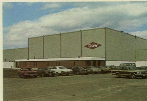
The Dow Chemical Company, Newark Ohio Industrial Park, Newark, Ohio. Architect: Curtis N. Lindberg, Columbus, Ohio. C-Panel System, Shadowwall Exterior Profile.
