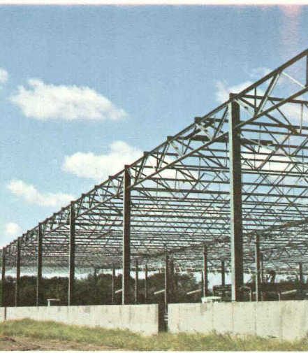
Joist girders have a simple span design. Which means why ponding calculations are easier. And design time is shortened.
