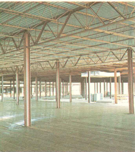
Joist girders need fewer foundations and columns. Which means less work for you and larger areas for your clients.
