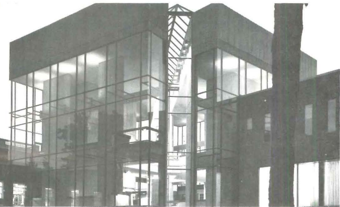
SHERMAN FAIRCHILD PHYSICAL SCIENCES CENTER , Hanover, New Hampshire. Jury Comments: "Handsome linkage of older existing buildings... greatly enhances whole... very effective functional solution." Owner: Dartmouth College, Hanover, New Hampshire. Architect: Shepley Bulfinch Richardson and Abbott, Architects, Boston, Mass. Structural Engineer: Nichols, Norton and Zaldastani, Inc., Boston, Mass. General Contractor: Jackson Construction Co., Boston, Mass.
