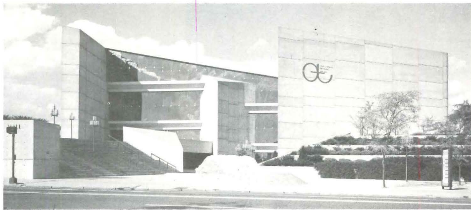
EDWIN J. THOMAS PERFORMING ARTS HALL , Akron, Ohio. Jury Comments: "Extremely competent in the planning and use of the site in a congested urban area... achieves human scale." Owner: University of Akron, Akron, Ohio. Architects: Caudill Rowlett Scott, Houston, New York, Los Angeles, Dalton, Van Dijk, Johnson & Partners, Cleveland, Ohio. Structural Engineer: R. M. Gensert and Associates, Cleveland, Ohio. General Contractor: Mosser Construction, Inc., Fremont, Ohio.
