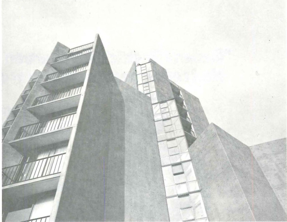
HOUSING FOR THE ELDERLY , San Francisco, California. Jury Comments: "Deft and imaginative... refreshing break from sterile box-like forms... nicely set into low-density urban site." Owner: San Francisco Housing Authority, San Francisco, Calif. Architect: Marquis and Stoller, Architects & Planners, San Francisco, Calif. Structural Engineer: Forell/Elsesser Engineers, Inc., San Francisco, Calif. General Contractor: The Pacific Co., Engineers & Builders, Berkeley, Calif.
