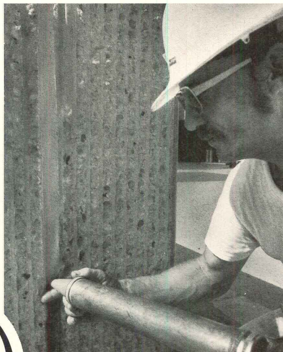
Applying an LP® polysulfide-base sealant.
