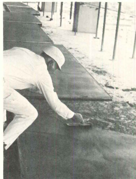
On-slab fabrication of the cement-plaster panels for the Hyatt Regency in Phoenix is shown above. With the mobility afforded by open floor space, it was possible for fabrication to proceed rapidly. Scratch coat has been applied in the photo above, left, and the finish coat is shown above, right.
