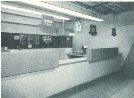
One of thirty-eight concession stands. Areas coated with Water Base Pitt-Glaze Acrylic-epoxy.
