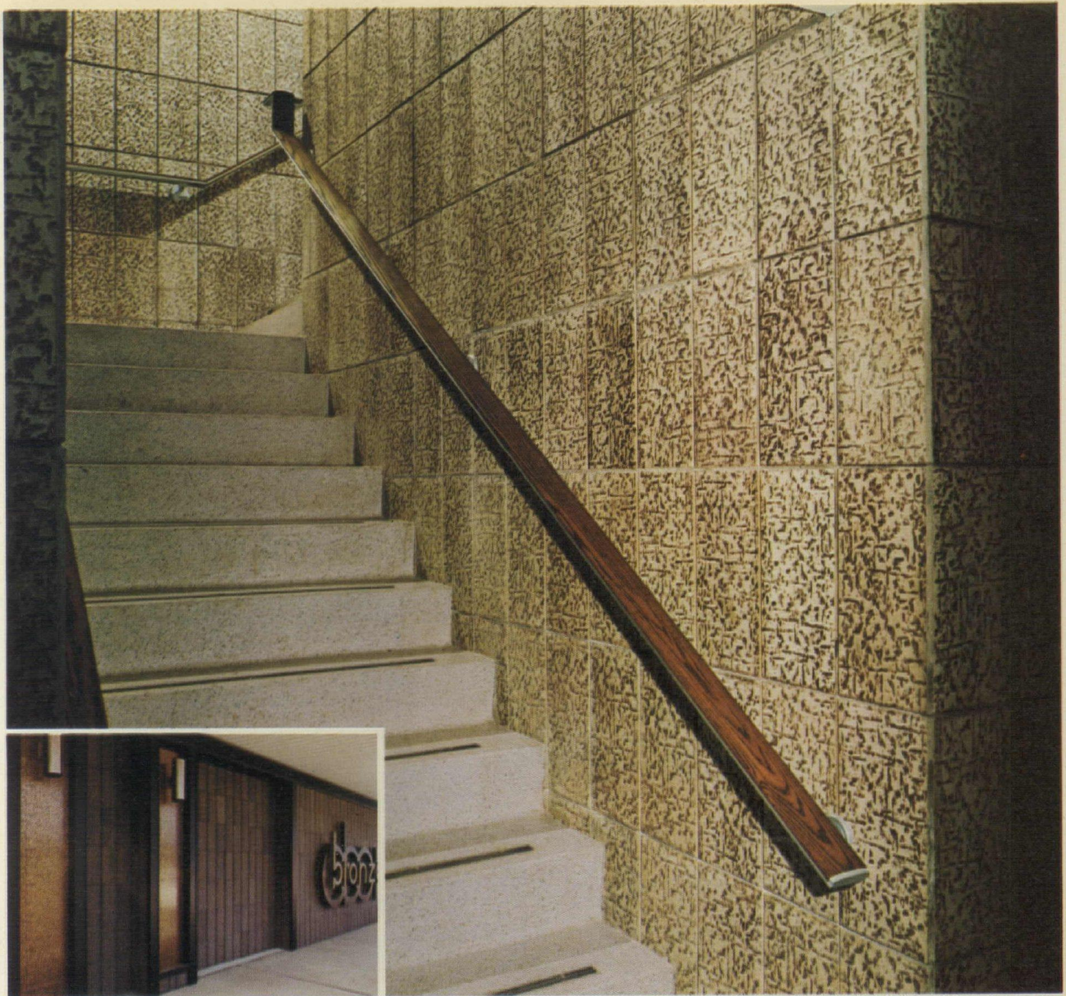
Interior and exterior installations of Stark textured tile.
