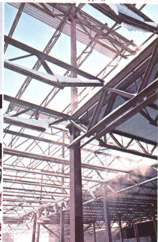
Joist girder design flexibility provided for a wide range of load support, from normal roof loads to heavy mechanical equipment loads.
