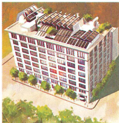
Printing House, New York City. Recycles an obsolete industrial building to create unique urban style housing. A vertical heat pump provides heating and cooling. Solar panels provide energy for domestic hot water. All insulation standards are upgraded. All windows are \frac{5}{8} -inch insulating glass.
