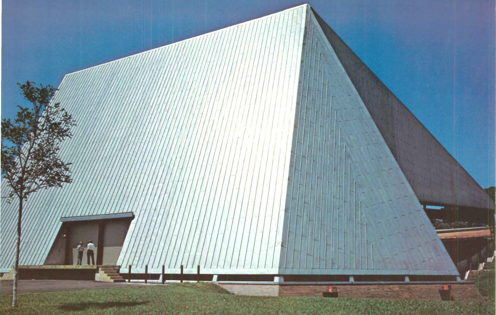
Robin Hood Dell West, Philadelphia, Pa. • Architects: John H. MacFadyen and Alfredo De Vido, New York • Associate Architect: I. Demchick, Philadelphia, Pa. • Roofing Contractor: Warren-Ehret-Linck, Philadelphia, Pa.
