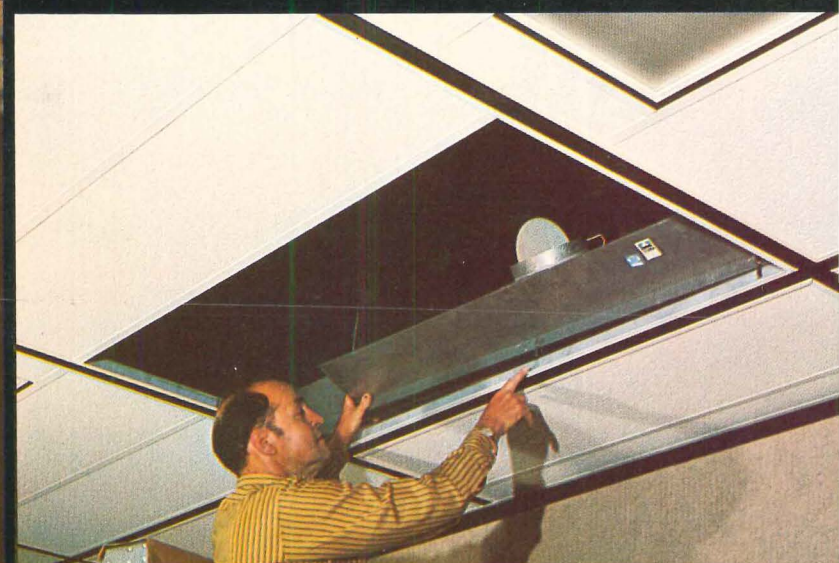
Air-handling options include air boot and bar for constant-volume systems as well as two variable-volume systems designed for energy savings.
