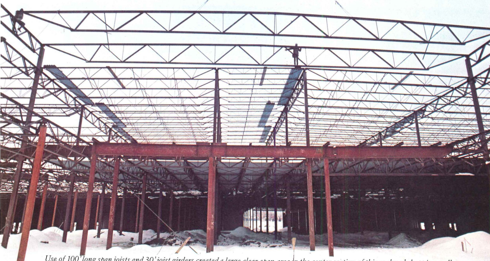
Use of 100' long span joists and 30' joist girders created a large clear span area in the center section of this enclosed shopping mall.
