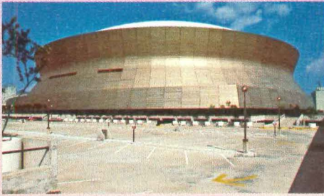
SUPER STADIUM: Superdome, a gleaming 500,000 sq. ft. expanse of Kalcolor aluminum, dominates the skyline of New Orleans.
