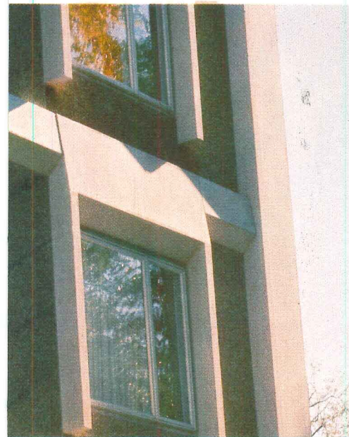
Cheesman Garden Apartments, Denver, Colorado Architect: Slater, Small & Spent; Denver Installation: Perma-Shield Casement operating and fixed units in precast frames
