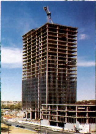
Ceco forming specialists formed a total of 834,000 square feet of flooring and averaged one completed 20,000 square foot floor every six working days.
