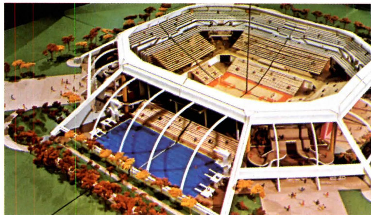
Permanent fabric exterior removed from model to illustrate column-free interior.
