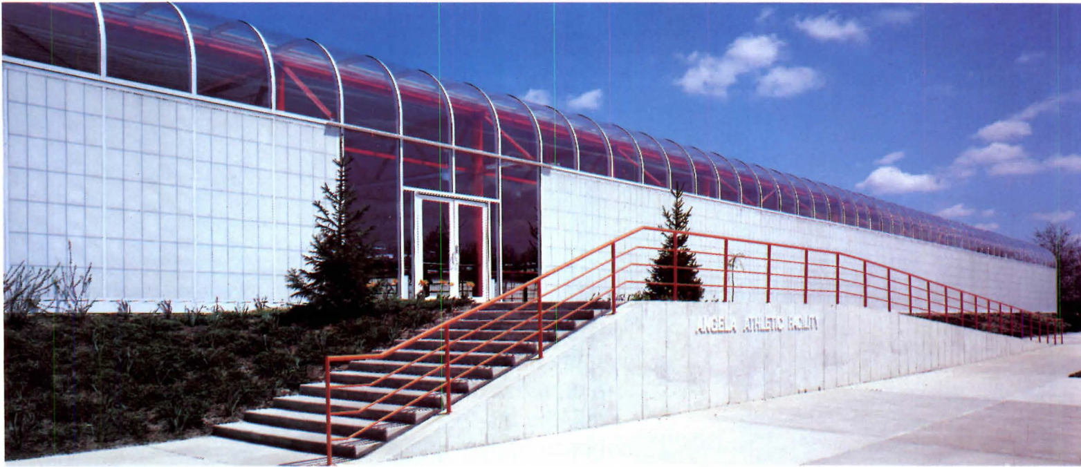
St. Mary's College C. F. Murphy Associates, Architects
