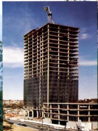
Ceco forming specialists formed a total of 834,000 square feet of flooring and averaged one completed 20,000 square foot floor every six working days.
