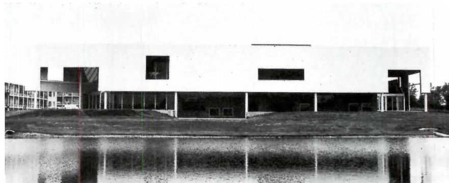
Completed Building: National College of Chiropractic Student Center, Lombard, Illinois; Hinds, Schroeder, Whitaker, architect. The jury admired the use of metal panels and found the design "a playful expression of an inert mass."
