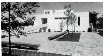
Completed Building: Savior Divine Lutheran Church, Palos Hills, Illinois; Jaeger, Kupritz Ltd., architect. With an "intimate quality," it "sets itself apart from neighbors and yet is not unfriendly."
