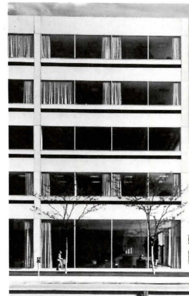
Completed Building: St. Joseph Valley Bank, Elkhart, Indiana; Skidmore, Owings & Merrill, architect. "A classic contemporary office building designed with particular care to the details," said the jury. "It is fresh in its expression."
