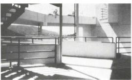
Planter boxes extend across the length of each floor, and also beyond the building in a series of bridges built with plywood box beams (photo opposite). As visualized by the architects in the rendering below, growth from the planters is intended to form an eventual camouflage over the entire building, and to contain the outdoor spaces.
