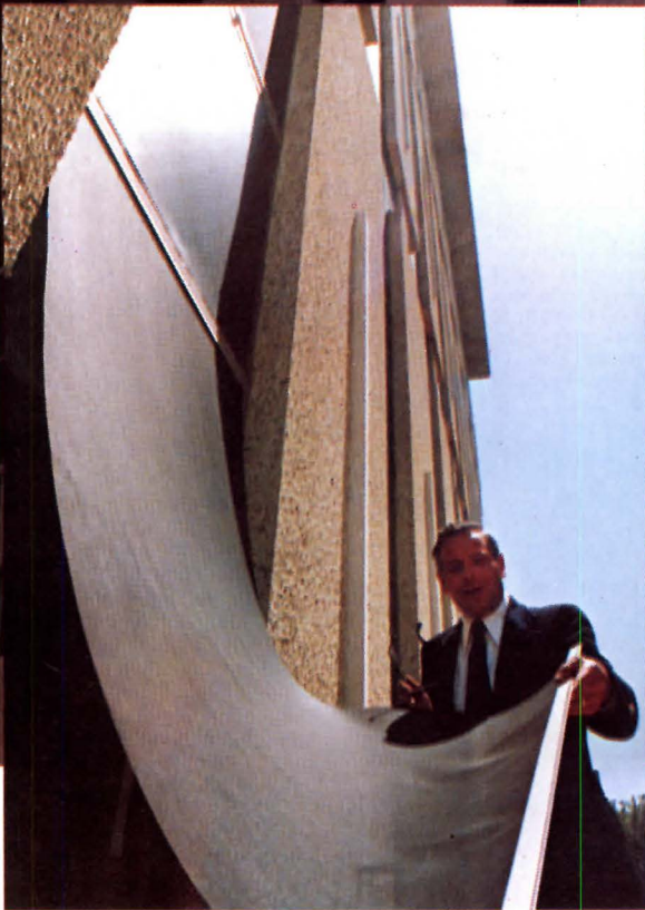
Phil Iatesta, Chief Engineer of Bethesda (Md.) Air Rights Building, shows how easily solar screen unlocks for window cleaning. He expects payback through energy savings in less than two years.
