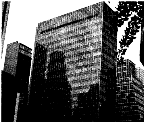
Lever House New York, New York, sealed with Thiokol polysulfide base sealant, 1954
