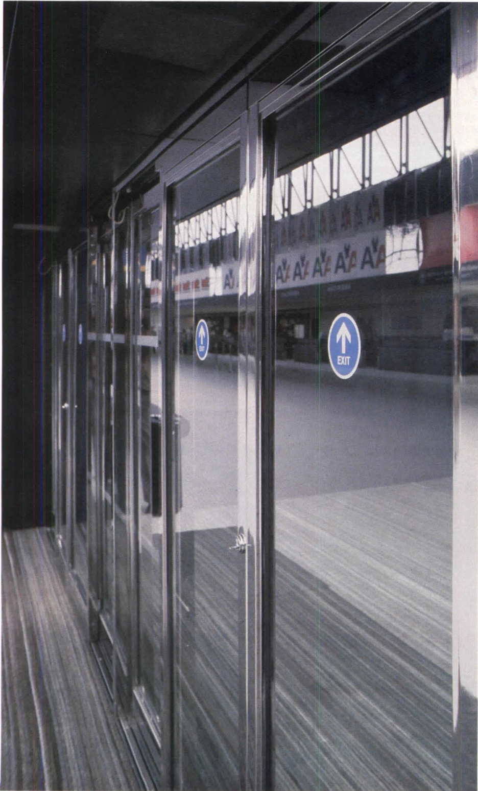
Sliding application with Stanley door hardware. Baltimore/Washington International Airport.
