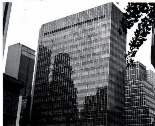
Lever House New York, New York, sealed with Thiokol polysulfide base sealant, 1954
