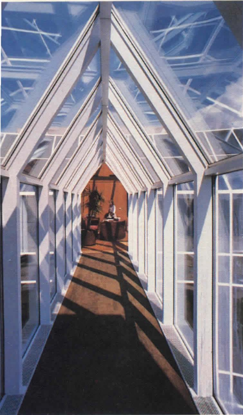
A steel-framed pedestrian bridge (above) connects the free-standing elevator tower to the garage, ground, and third levels. The concave facade (left) emphasizes the entrance and preserves as much of the landscape as possible.
