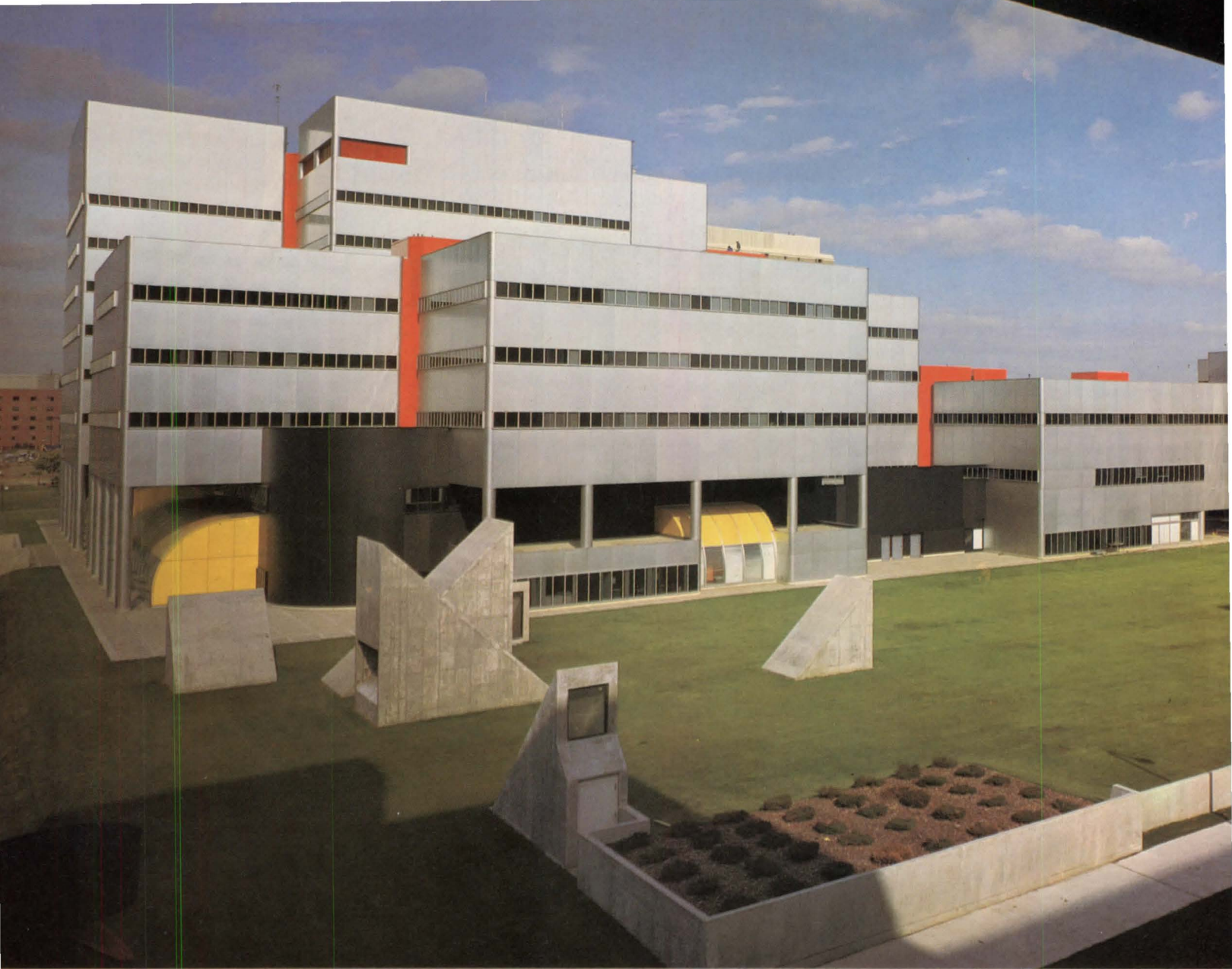
Giant concrete pyramids function as periscopes and light wells for an underground tunnel system connecting the various hospitals in the complex. The large black anodized aluminum cylinders serve as air intakes for a 630-car underground garage and the hospital. The yellow vaults serve to visually bridge the distance between building and site.
