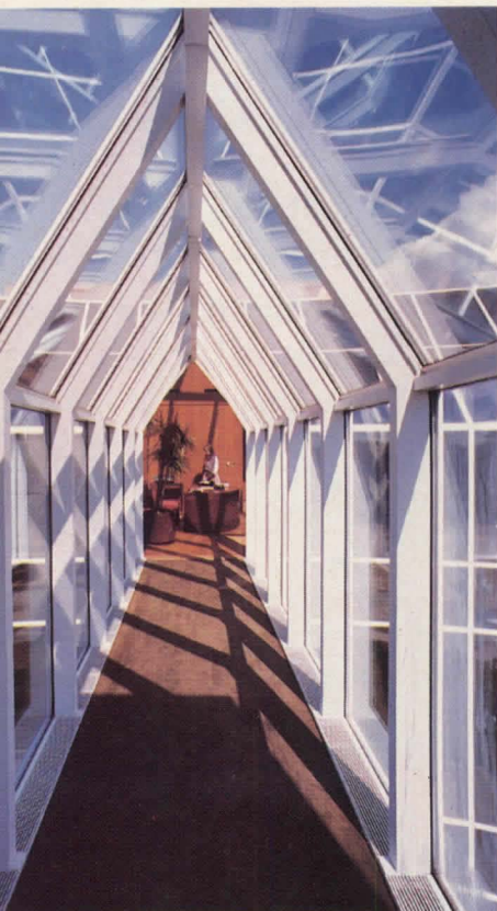
A steel-framed pedestrian bridge (above) connects the free-standing elevator tower to the garage, ground, and third levels. The concave facade (left) emphasizes the entrance and preserves as much of the landscape as possible.
