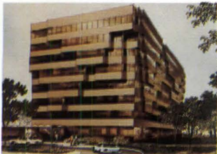
Greenspoint I, Houston, TX Arch: S.I. Morris Engr: Walter P. Moore & Co. Cont: McGregor Construction Co. Dvlpr: Friendswood Development Co. (Exxon)
