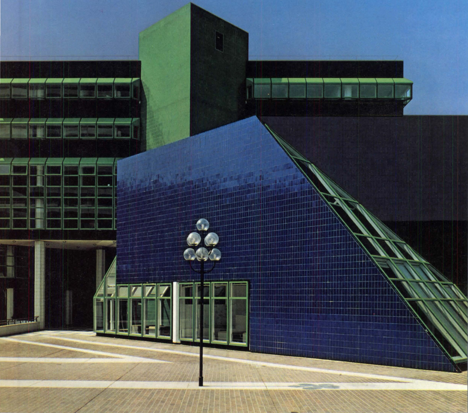
Cergy Pontoise Hotel, near Paris, clad in Monocolor #144 Intensive Blue and #143 Intensive Green. (Thin-set latex mortar on precast concrete. Architects: Claude Vasconi and Georges Pencreach.
