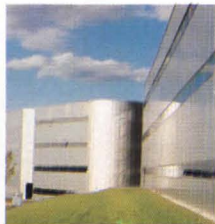
GTE/Hines, Westboro, MA Arch: Drummey, Rosane, Anderson Engr: Anderson-Nichols & Co. Cont: Vappie & Co., Inc.
