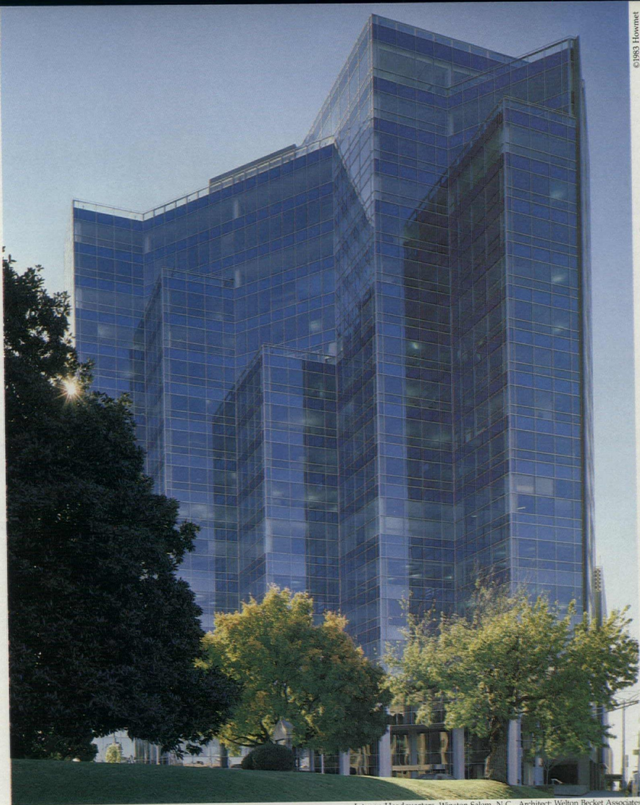
Intagon Headquarters, Winston-Salem, N.C., Architect: Welton Becket Associates
