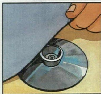
1 Roll membrane over knobbed base plate.
