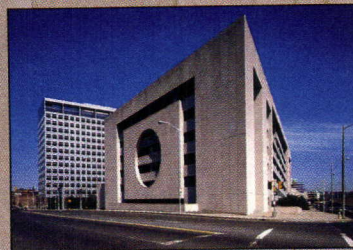
A site-cast concrete parking garage formed by Ceco.
