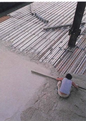
Composite deck simplifies construction
