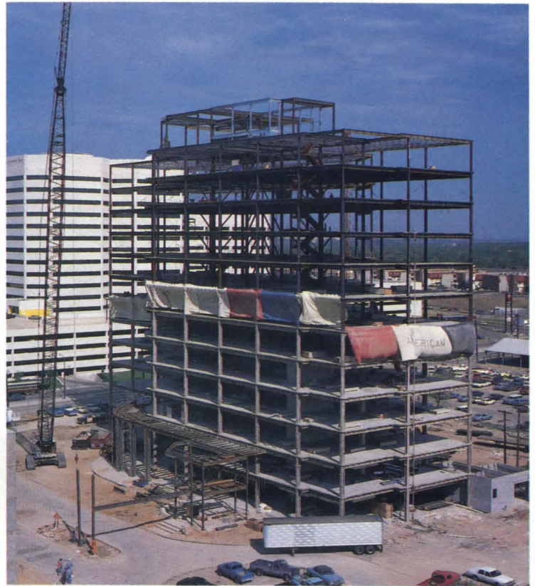
Vulcraft deliveries eliminated "lay down space" worries
