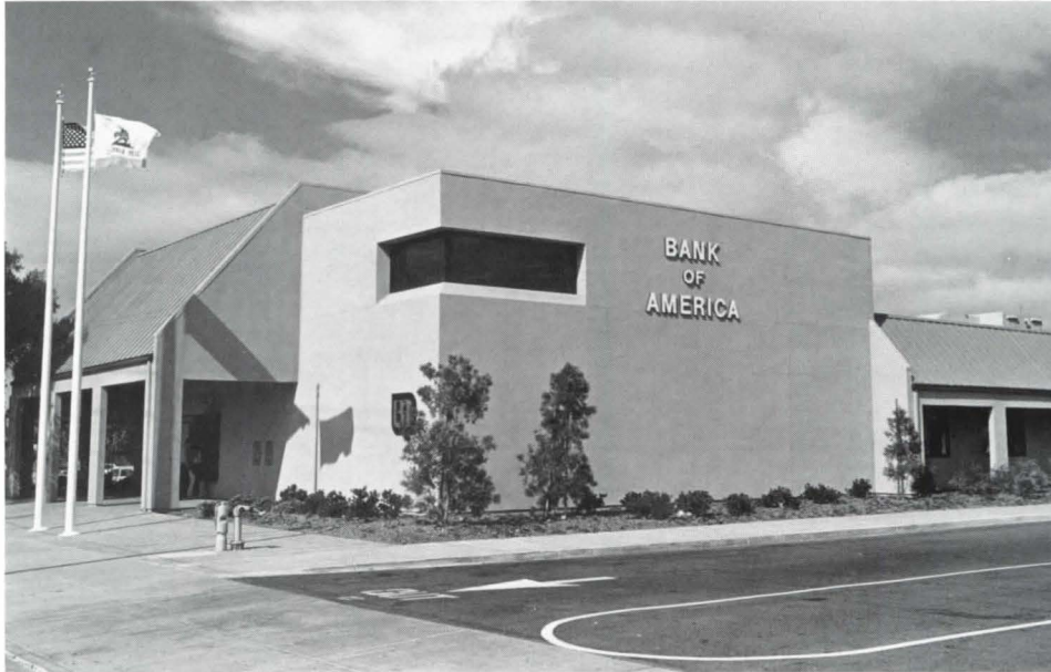
Conventional exterior of Bank of America's Livermore branch uses novel cooling system based on ice bank storage.
