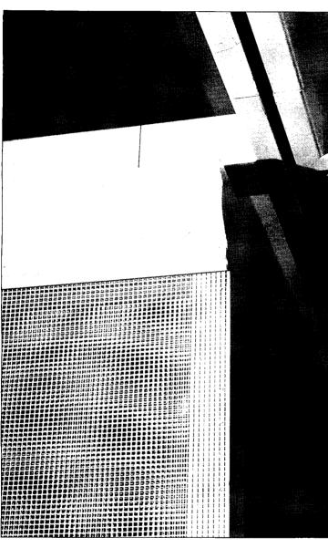
Though formed of seemingly simple, familiar hardware that might have come from the shelves of the local building-supply house—steel-framed perforated-metal panels suspended from an overhead channel/grid—SITE's floating wall system achieves refinement through painstaking engineering and craftsmanship, abetted by classical cornice and base moldings that recall the historic roots of its setting.
