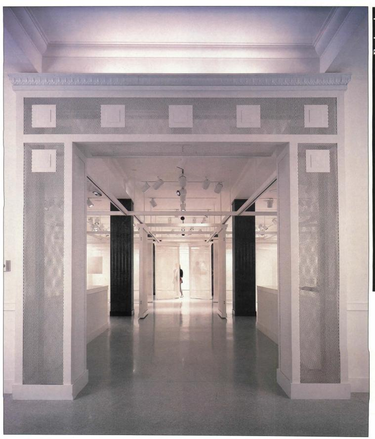
A repertoire of eight patterns of round or square perforations and the ability to mount different perforation patterns on either side of each wall section yield almost unlimited variations in background density to complement displays. At the extremes, complete transparency is made possible by a picture molding that allows hung objects to float in an empty frame, while complete opacity can be achieved by
