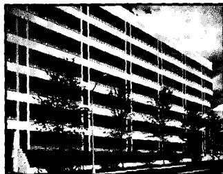
1275 Peachtree at the Circle Atlanta, Georgia Thompson, Ventulett, Stainback & Associates
