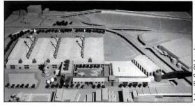
Inc., of Columbus (lower left) -a high-tech Brobdingnagian structure that called for 24-footdeep steel trusses spanning 270 feet and set on 120-foot centers.
