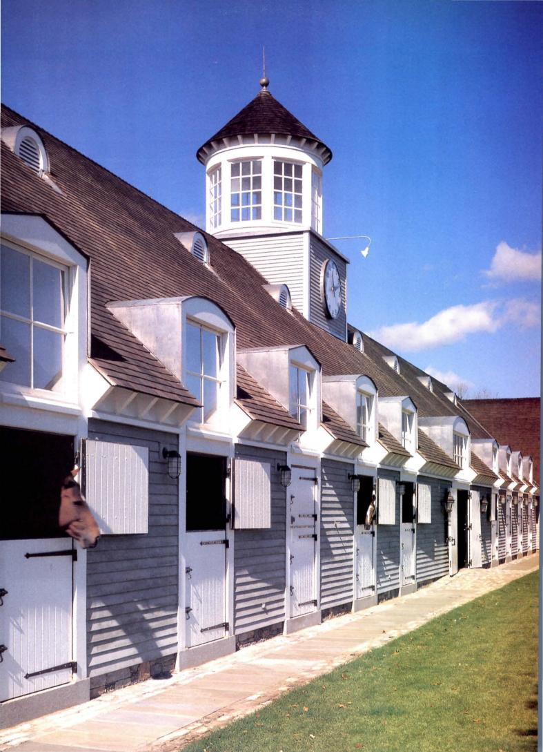
Both the forthrightness and the elegance of the stable complex's exteriors carry through to its interiors. A hybrid stable plan, providing both a central corridor and direct access from stalls to the outside, joins with doors and dormers to admit plentiful light and ventilation.
