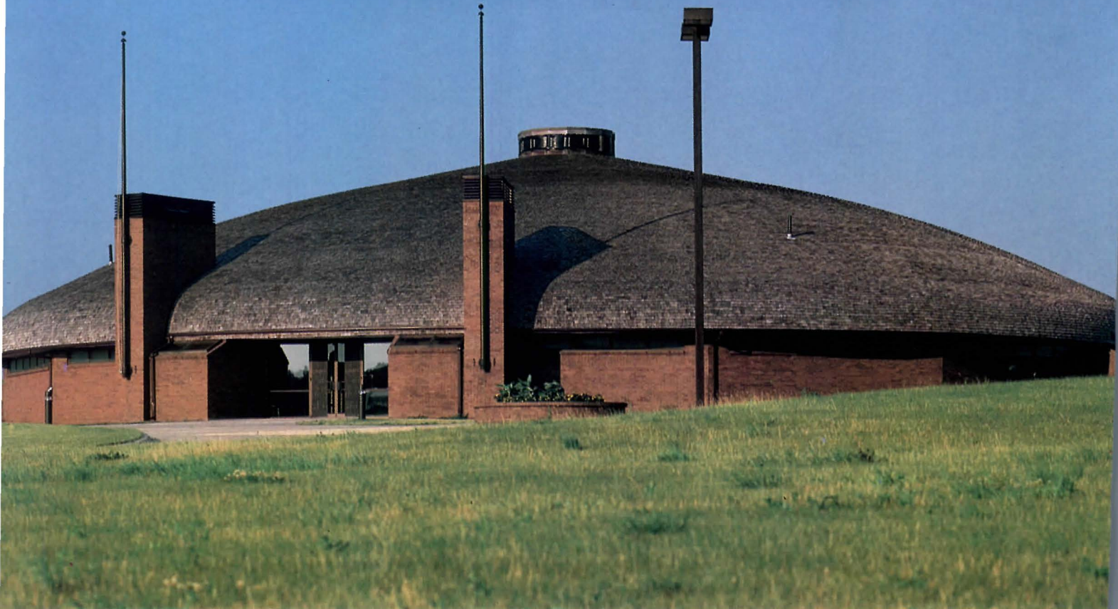
Architect: Voorhees Design Group, Inc.
