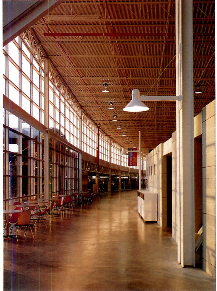
Above: Two views of the “street” that unites manufacturing (left in left photo, right in right photo) and office areas.
