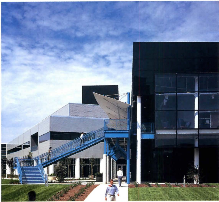
A canopied entry and black-glass cladding distinguish the fitness and training area from the rest of the metal-sided building (above left and top). An entry in striped concrete (right) evokes adjacent buildings.
