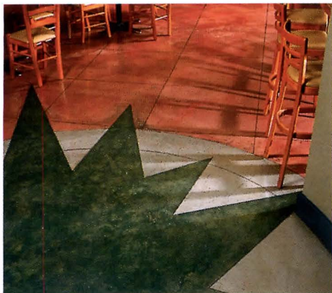
Bold graphic on a restaurant floor is an integrally colored concrete overlay of an existing slab, finished with a clear sealer.
