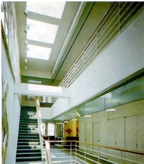
At the NRDC Building, the Croxton Collaborative brought daylight in from a skylit atrium (left). At Audubon House, the firm used glass partitions to allow sunlight to penetrate deep into the offices (below).
