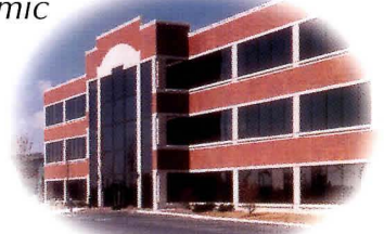
Professional Services Building, Allentown, PA
