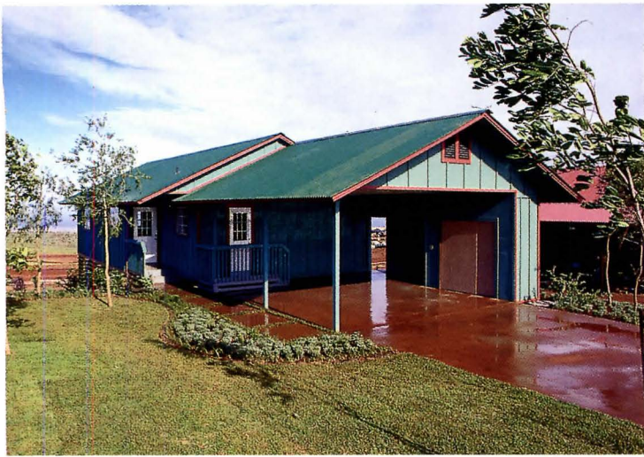
A low-budget use of colored concrete: the drive and walkway of a Hawaiian bungalow are tinted to blend with the red volcanic soil.
